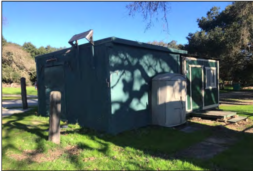
Photograph 3: Saddle dressing shed (right) and attached storage shed (left), looking northwest.
