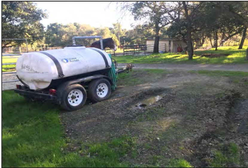
Photograph 7: Portable water storage tank with gas-powered pump, looking northeast. A small pool of liquid is next to the tank.
