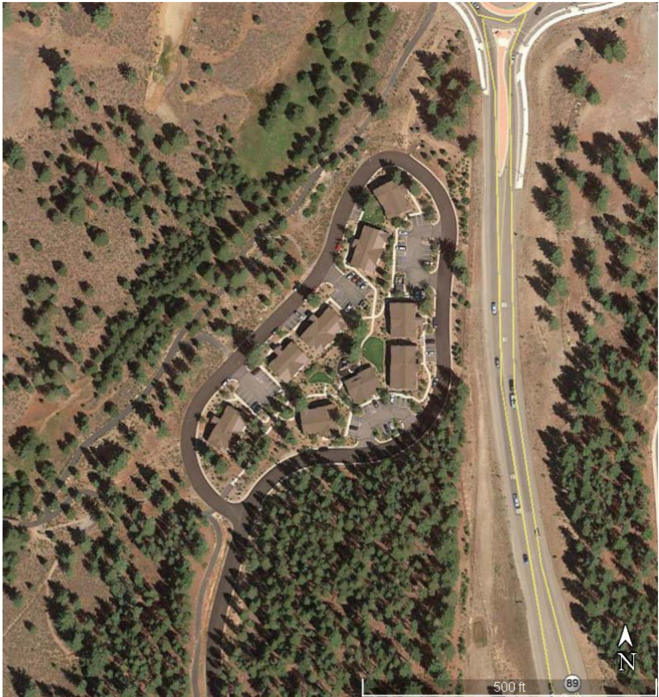
Figure 2. Google Earth July 2018 Image of the Site and Adjacent Areas. (Note This was taken after Phase 1 was built.)
