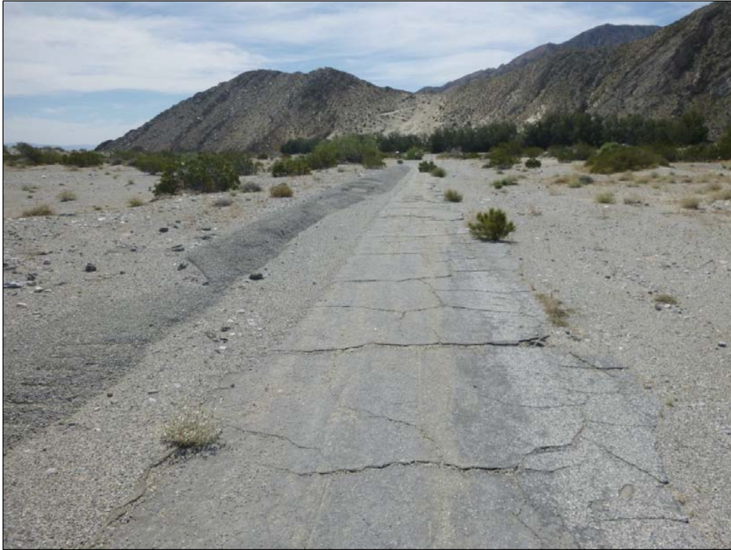
Figure 8 Overview of CA-RIV-12628H (view to the southeast).
