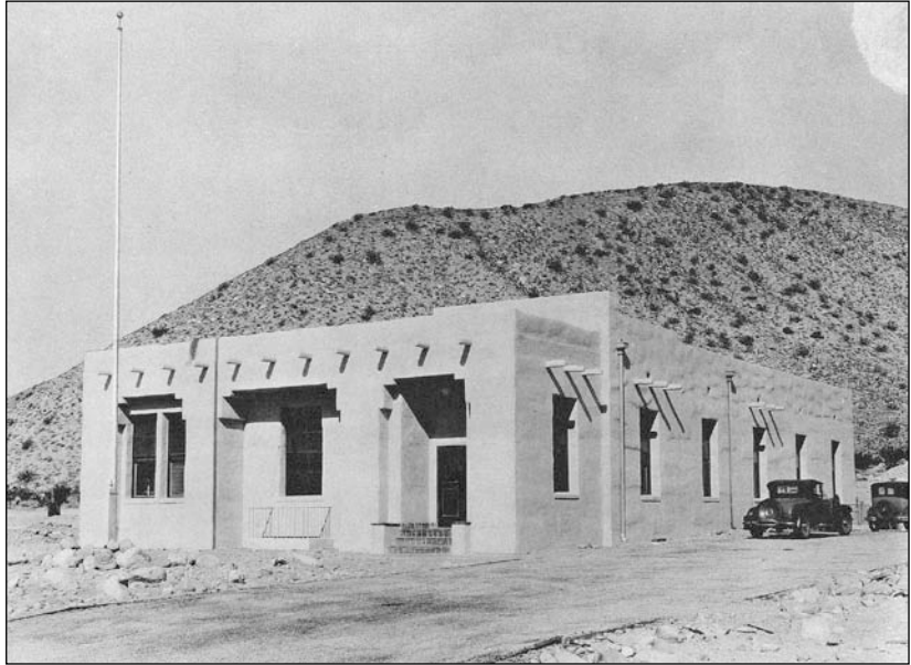
Figure 3 Whitewater Repeater Station, 1930 (Courtesy of AT&T Archives and History Center).
