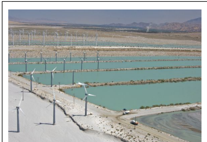
The Facility is located within the City of Palm Springs in Riverside County. This Facility consists of 19 replenishment ponds used to receive imported Colorado River water and natural inflows.
