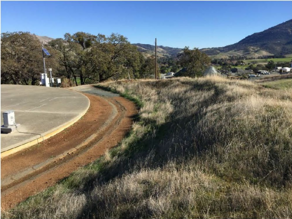
Photograph 1: Murchio Reservoir at left on parcel APN 122-020-006. A portion of the active quarry is shown at right.
