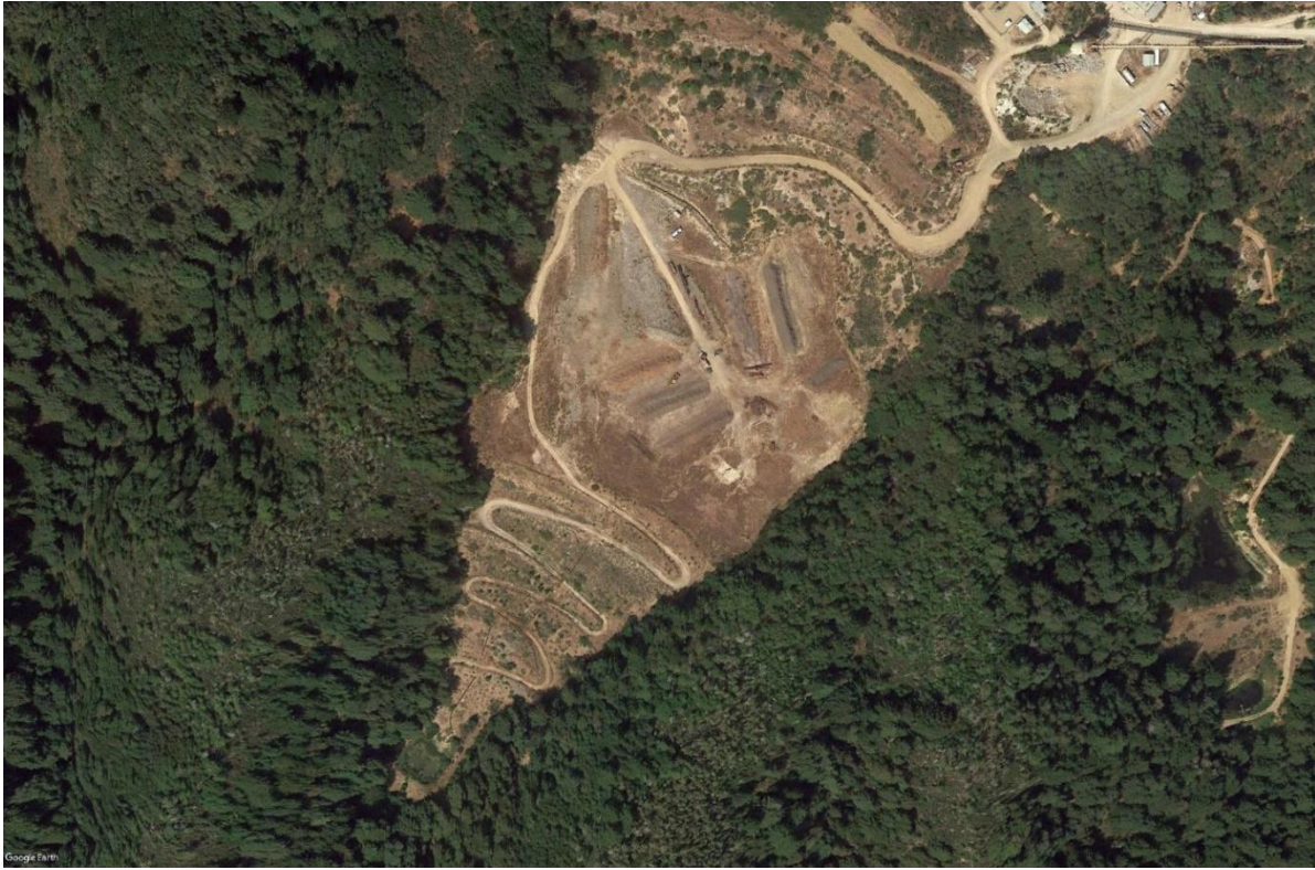
Figure 3.10-1. Limestone and marble quarry tailings pile in Liddell Creek watershed. Lat. 37.022618, Lon. -122.157659.
