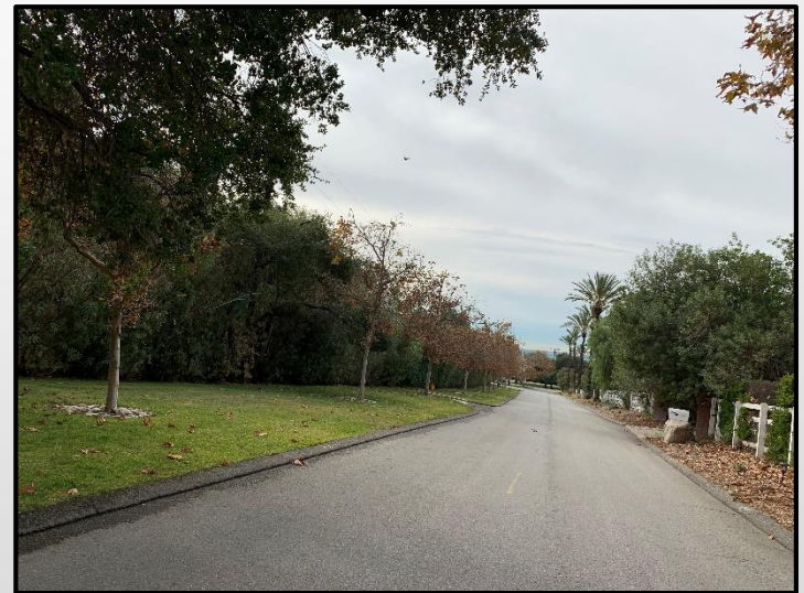
Photograph 20. Photograph of existing Bliss Canyon Road. Photograph facing south towards intersection with Deodar Lane.
