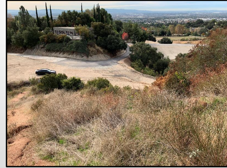
Photograph 12. Photograph looking south towards the existing Flood Control Road and Bradbury Debris Basin at the entrance of the Project site. Note this is the location where the looped Flood Control Road will intersect.
