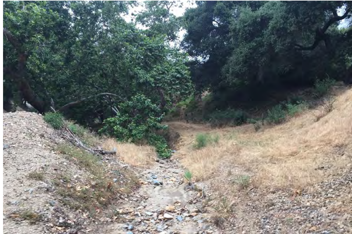
Photograph 5. View from the southern portion of the offsite improvement area looking at Drainage B.
