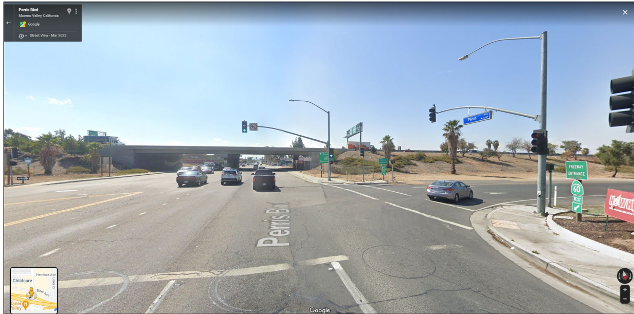
Figure 2-5: Perris Boulevard at State Route 60, view looking south
