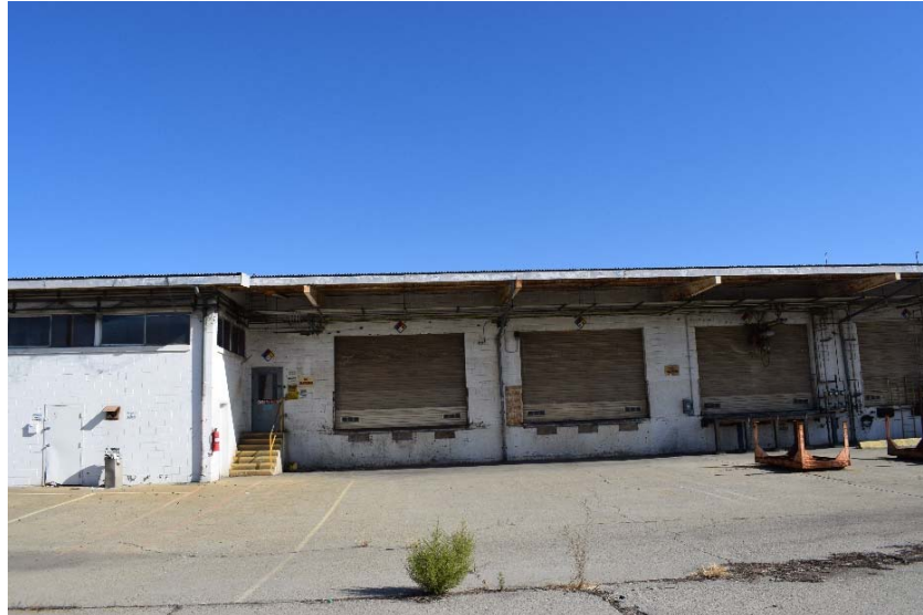
Figure 6. Compressed gas plant, south façade, facing north, October 10, 2019. Source: ICF.
