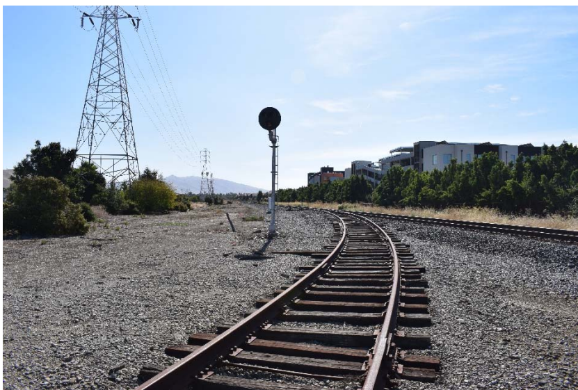
Figure 9. SPRR spur (foreground) and SPRR main line (background), facing southeast, October 10, 2019. Source: ICF.
