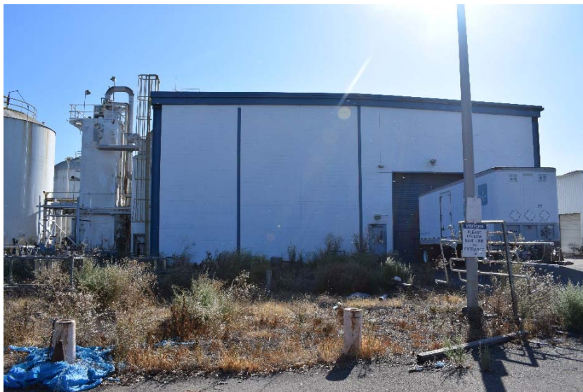
Figure 8. Air separation plant/compressor house, west façade, facing east, October 10, 2019. Source: ICF.
