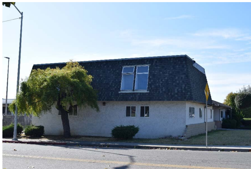
Figure 5. Office building's north façade, facing south, October 10, 2019. Source: ICF.
