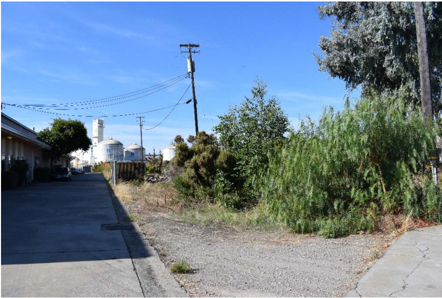
Figure 2. North portion of Line 1 at 7 th Street, looking southwest. Tracks are not visible from public right of way because of overgrown vegetation and private parcel access. Source: ICF, October 10, 2019.
