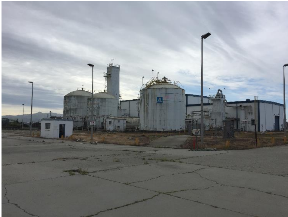
Photograph 6. Developed land with no trees in the northern portion of the project site. Facing west.
