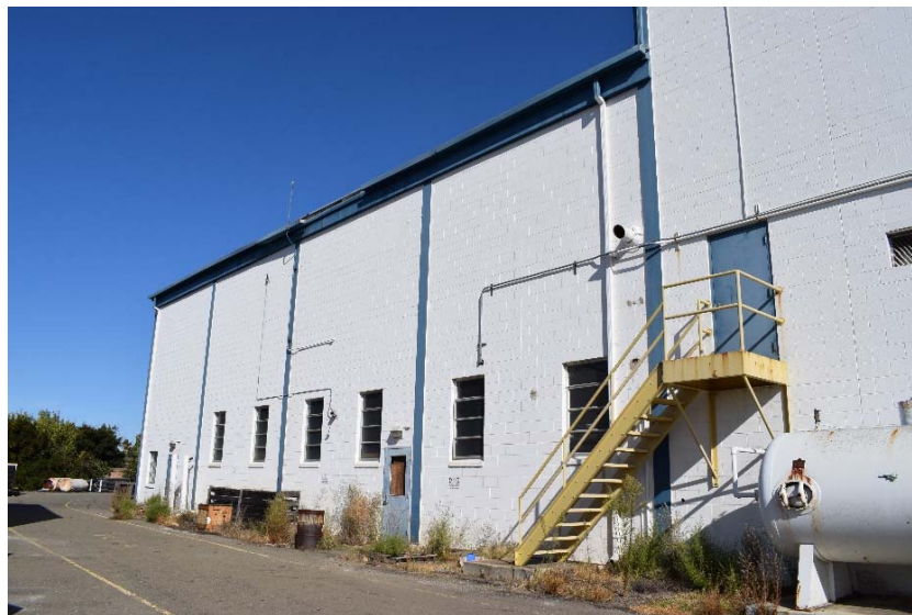
Figure 7. Air separation plant/compressor house, south façade, facing north, October 10, 2019. Source: ICF.
