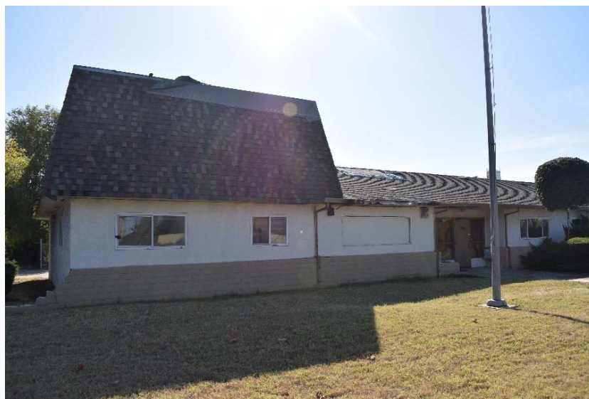
Figure 3. Office building at the industrial plant's northwest corner, facing east, October 10, 2019. Source: ICF.
