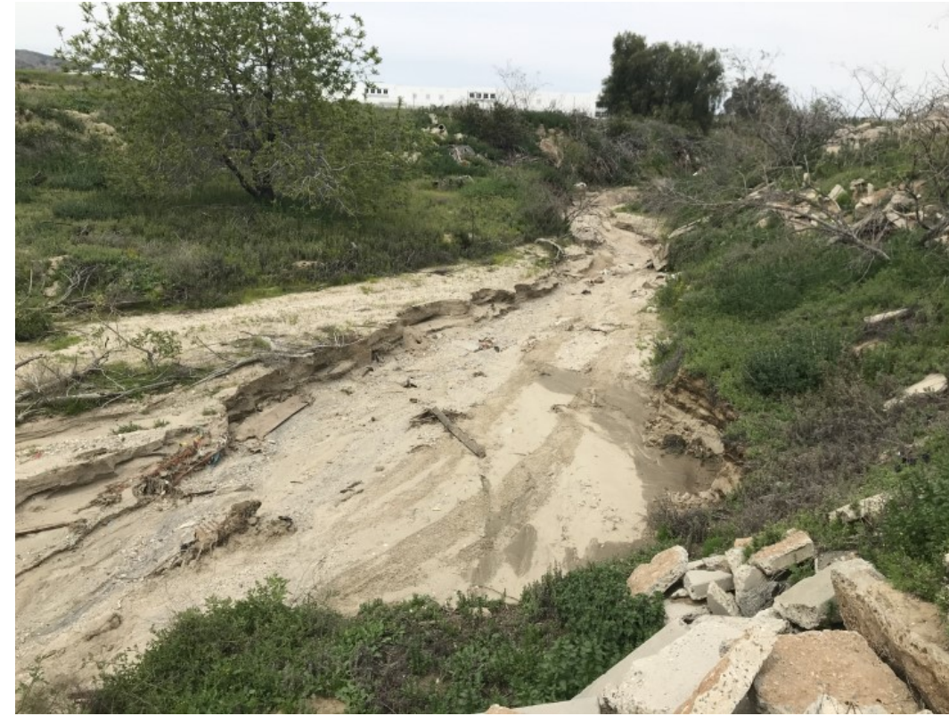
Photograph 2: 03-31-20. South-central portion of Quincy Channel looking north.
