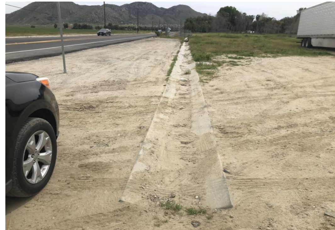
Photograph 8: 03-31-20. View of non-jurisdictional v-ditch constructed in the uplands.
