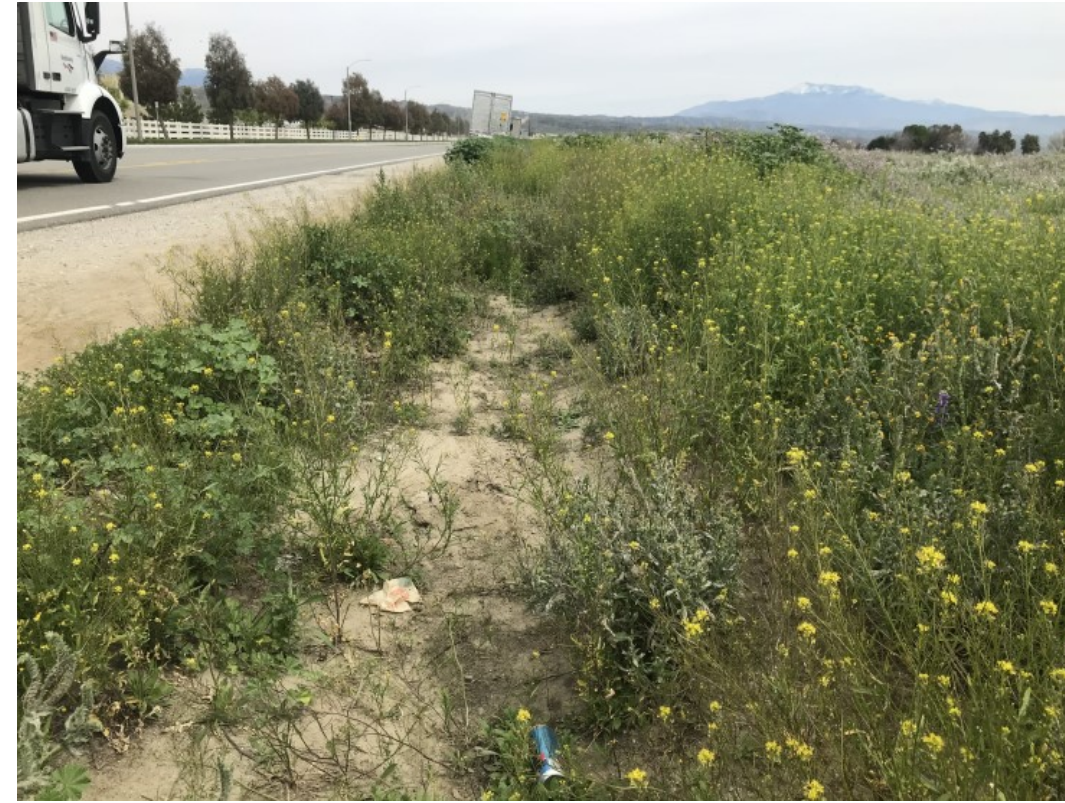
Photograph 6: 03-31-20. Representative view of roadside ditch looking east.
