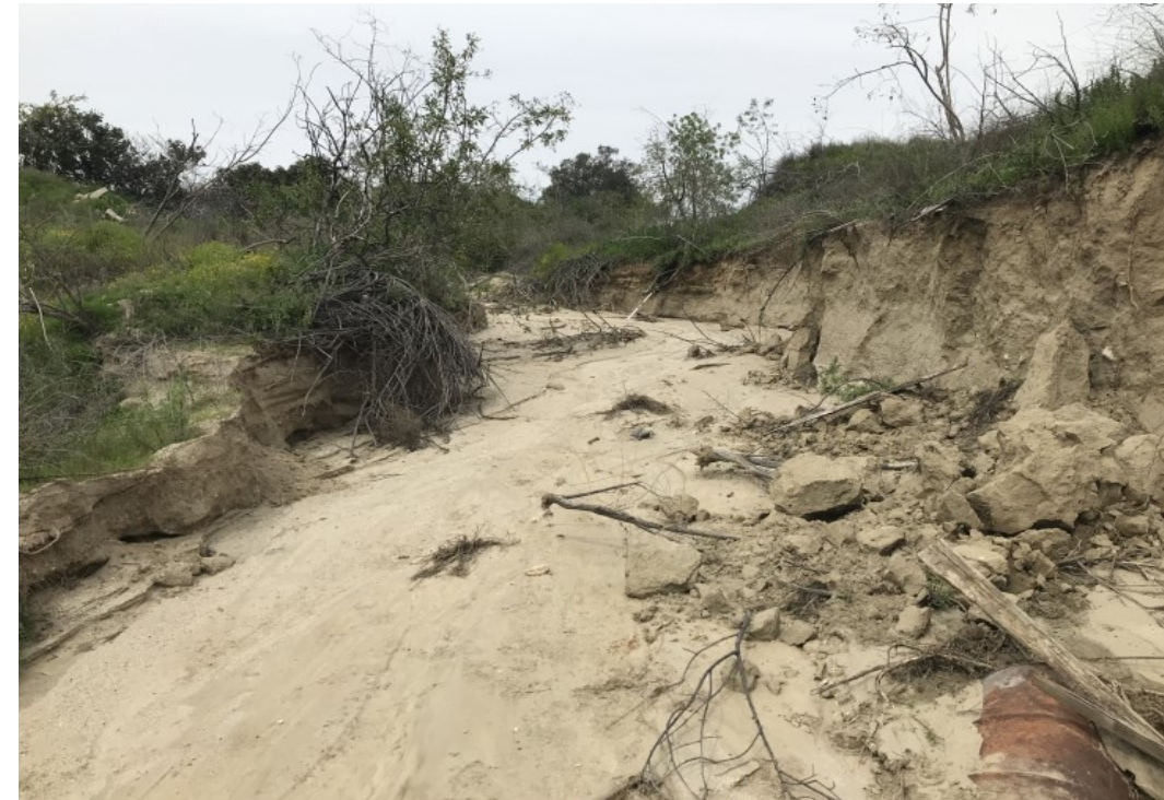
Photograph 4: 03-31-20. Additional view of Quincy Channel looking north.
