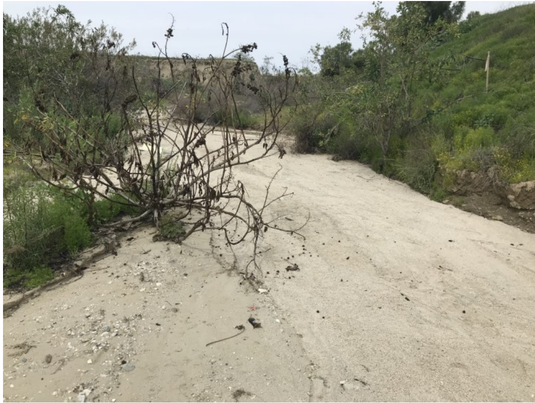
Photograph 1: 03-31-20. Southern portion of Quincy Channel looking north.
