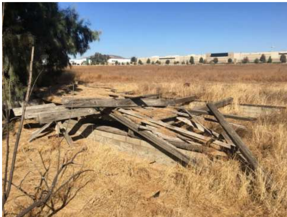
Figure 5 Building Foundations, View to Northwest
