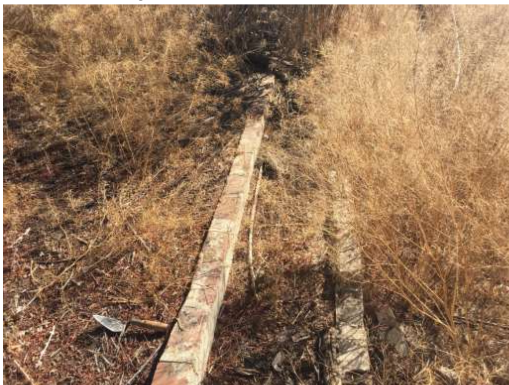
Figure 6 Brick-Lined Trough, View to East
