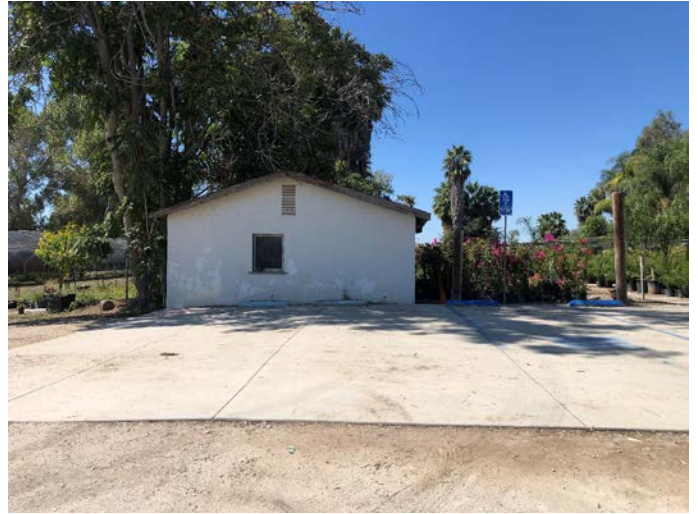
East Elevation of Garage
