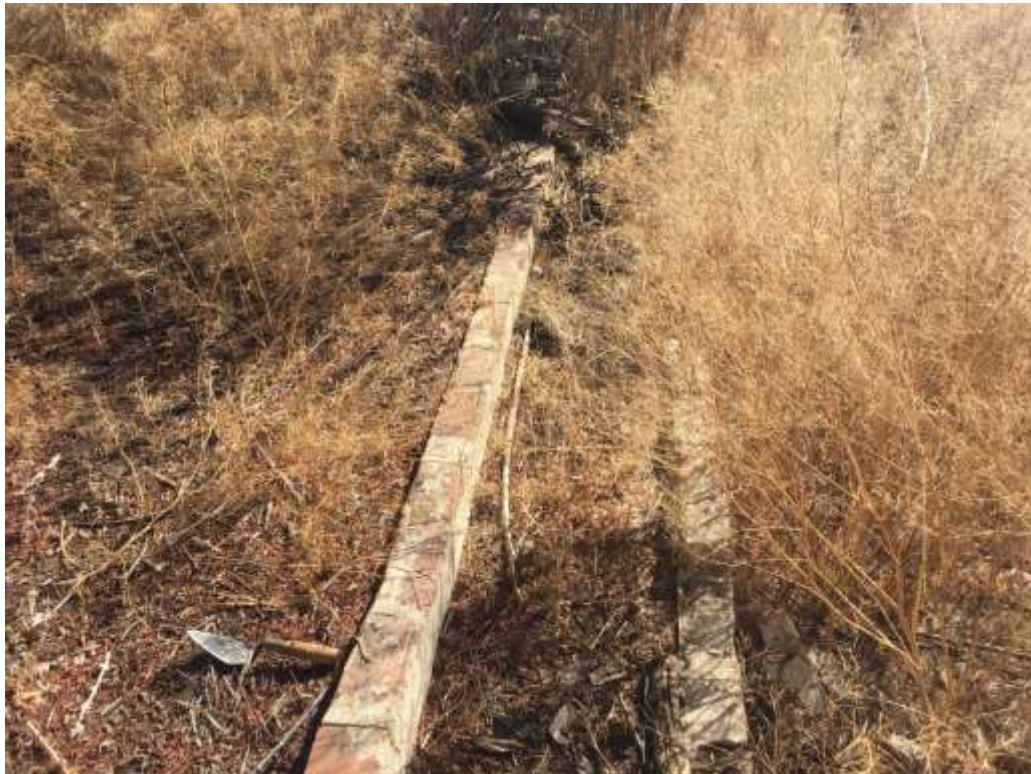
Photograph 2. Brick-Lined Trough, View to East
