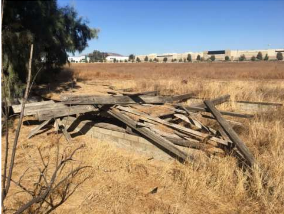
Photograph 1. Building Foundations, View to Northwest
