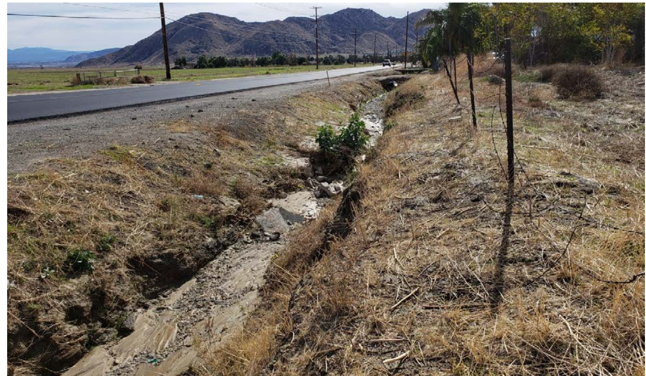
Photograph 4: Photo of Drainage Ditch 2 running parallel to Redlands Boulevard. Note the lack of vegetation.
