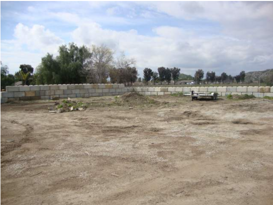
PHOTO 39 VIEW OF THE LARGE CONCRETE BLOCK AT THE WEST-CENTER PORTION OF THE PROPERTY. THE CONCRETE BLOCK ARE THE START OF BUNKERS FOR SAND GRAVEL AND ROCK.
