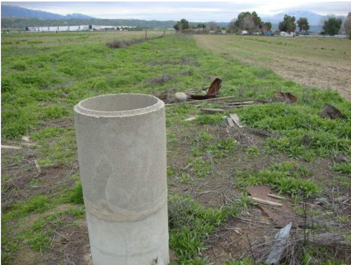
PHOTO 17 VIEW FACING EAST FROM THE INTERSECTION OF PARCELS 002, 003, 009 AND 010 SHOWING THE IRRIGATION STANDPIPE IN THIS AREA AND REMNANT FENCING. SHEET METAL AND WOOD FROM PRIOR STRUCTURES IS ALSO VISIBLE. HALLS NURSERY IS IN THE BACKGROUND.
