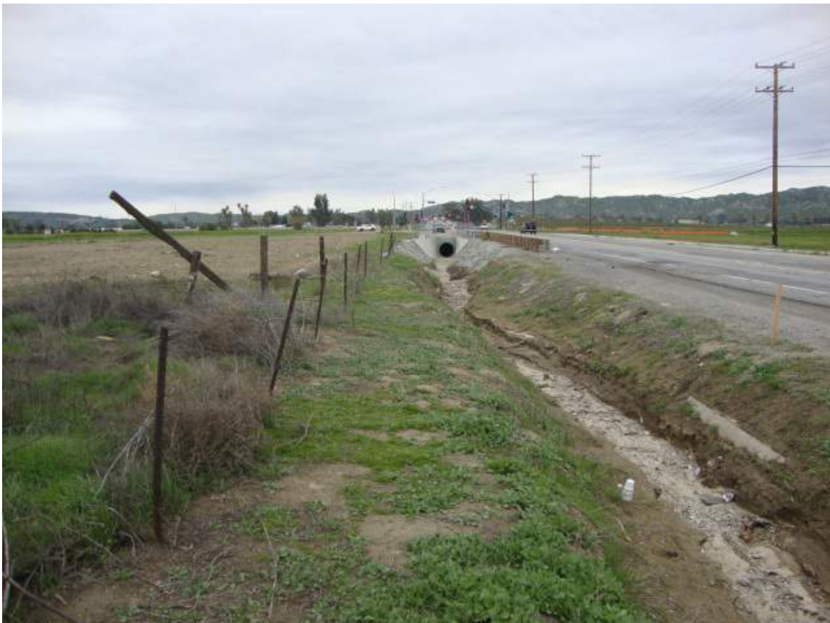
PHOTO 4 VIEW FACING NORTH FROM THE SEC OF PARCEL 004 SHOWING THE SITE TO THE LEFT (WEST) WITH REMNANT FENCING. REDLANDS BLVD. IS PRESENT TO THE RIGHT WITH THE CONCRETE AND EARTHEN DRAINAGE VISIBLE.
