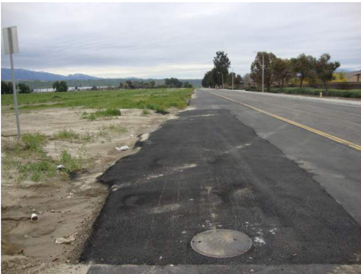
PHOTO 12 VIEW FACING EAST FROM THE SWC OF PARCEL 011 SHOWING THE SITE TO THE LEFT (NORTH) AND ENCELIA AVE. AND SINGLE FAMILY RESIDENTIAL TO THE RIGHT. A SEWER MANHOLE IS VISIBLE IN THE FOREGROUND.
