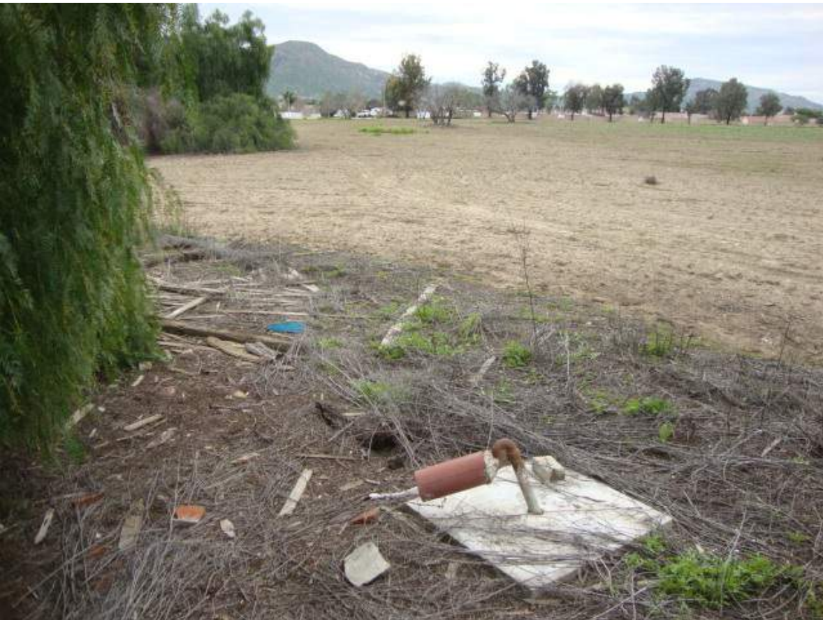
PHOTO 20 VIEW OF A WELL REPORTED IN PREVIOUS ENVIRONMENTAL STUDIES FOR THE SITE LOCATED ON THE WEST SIDE OF THE PEPPER TREES AT THE INTERSECTION OF PARCELS 002, 003, 009 AND 010. THE PIPE IS APPROXIMATELY 2 INCHES IN DIAMETER AND THE CONCRETE IS APPROXIMATELY 2 FEET SQUARE. THE PIPE IS LOOSE AND CAPPED WITH CLAY PIPE AND CONCRETE.
