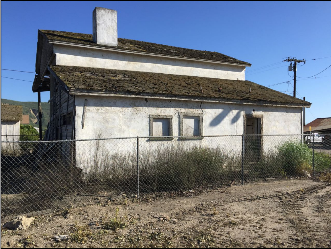
Photo 3. More-Edwards Adobe, northern elevation [3-31-17].
