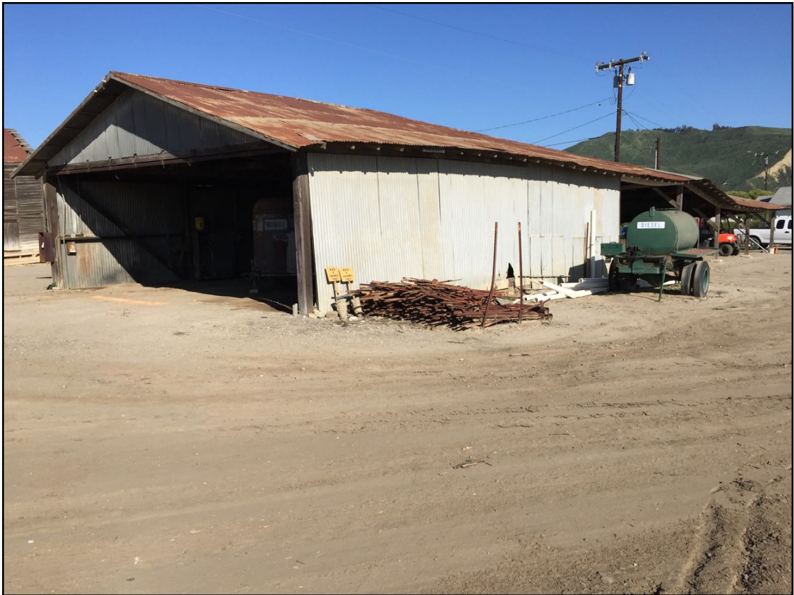
Photo 10. Equipment sheds, southern and western elevations. [3-31-17]
