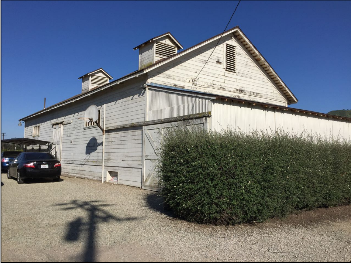
Photo 11. Barn, southern and western elevations. [3-31-17]
