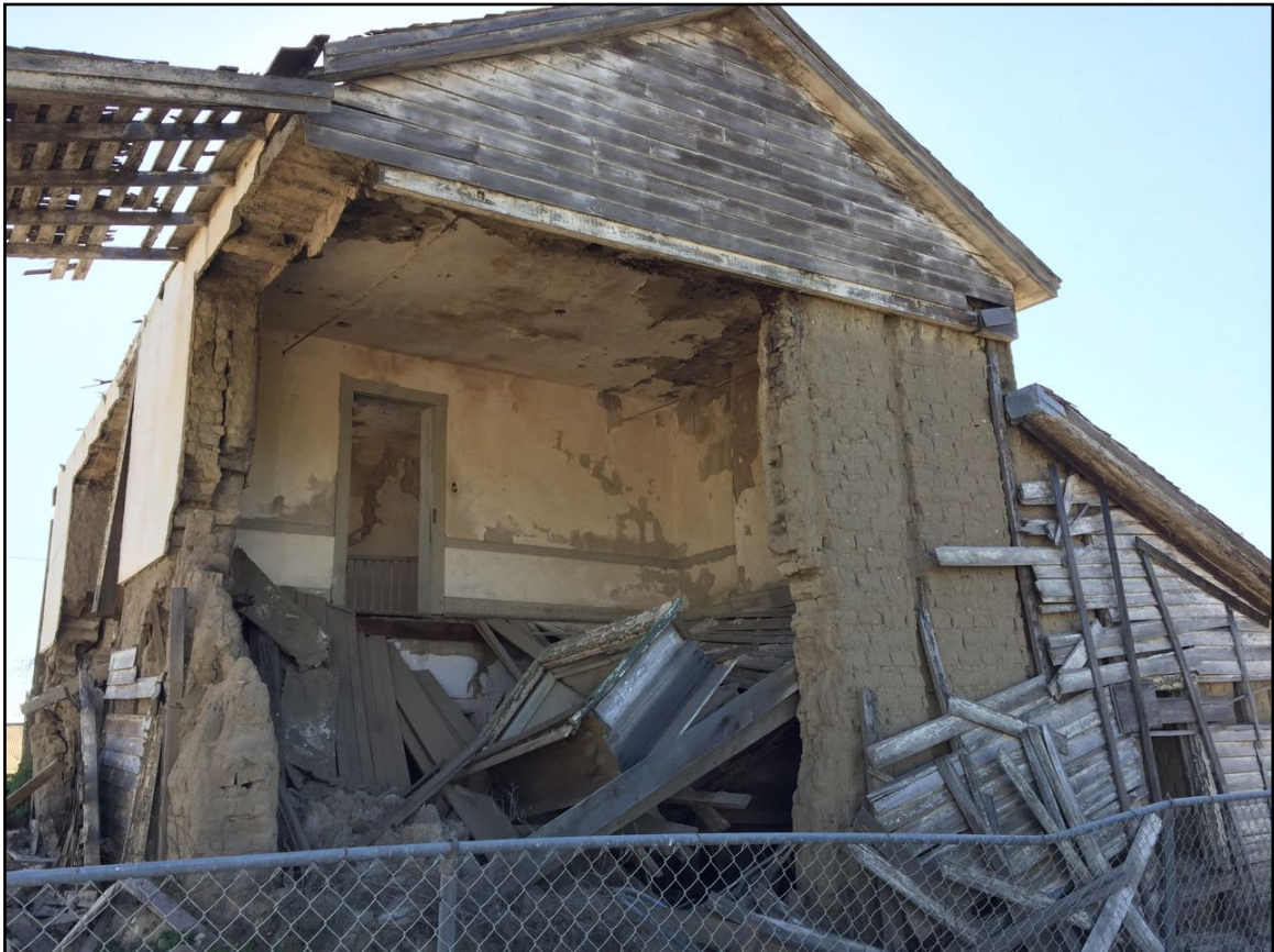
Photo 2. More-Edwards Adobe, eastern elevation. [3-31-17]
