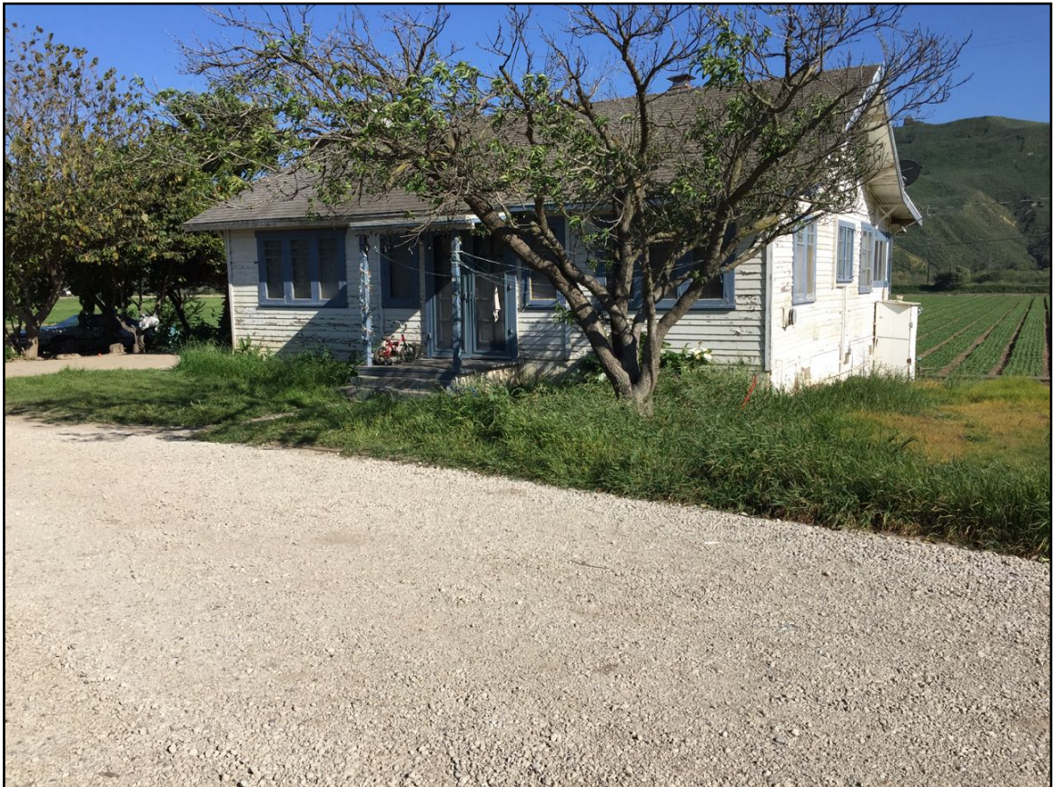
Photo 14. Ranch Residence, northern and western elevations. [3-31-17]
