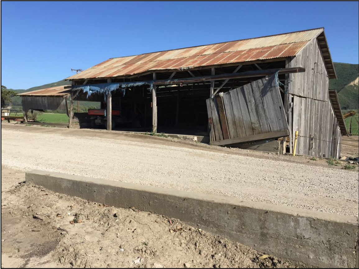
Photo 15. Barn, northern and western elevations. [3-31-17]
