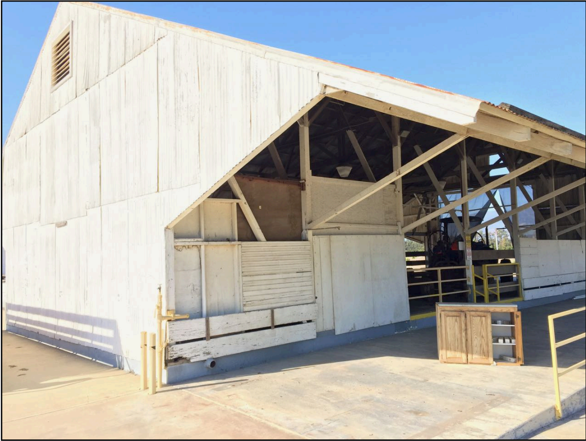
Photo 13. Equipment Shed, southern and eastern elevations. [3-31-17]
