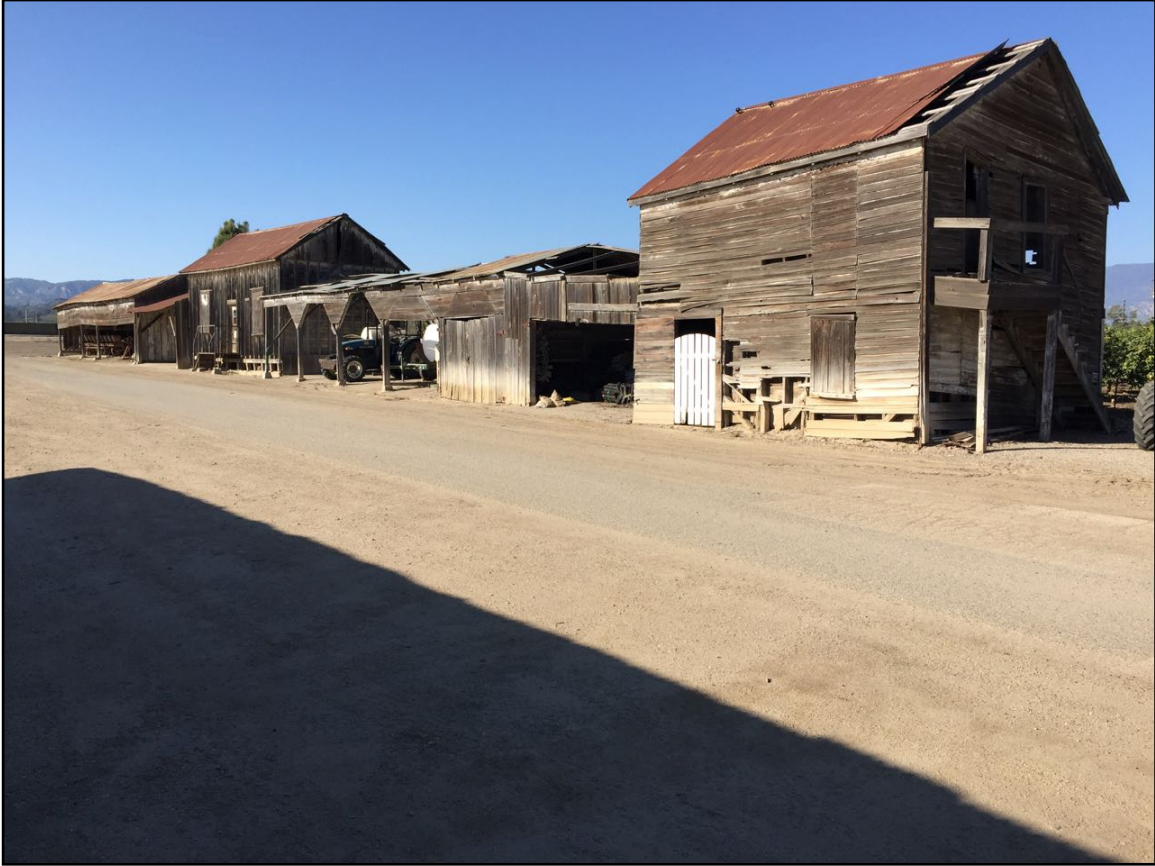
Photo 5. Barns and schoolhouse, western elevation. [3-31-17]
