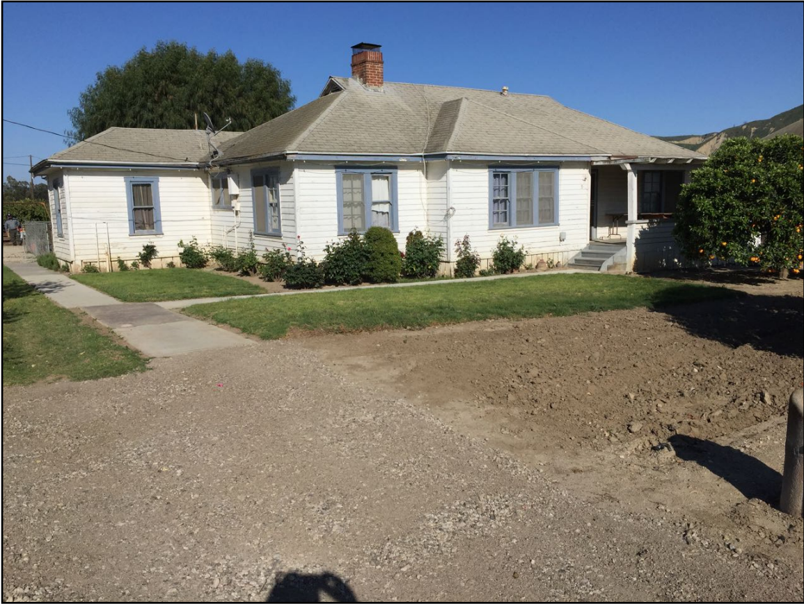
Photo 7. Residence, western elevation. [3-31-17]
