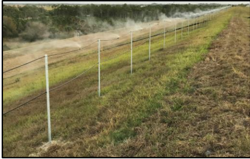
FogCo installed along fence line.
