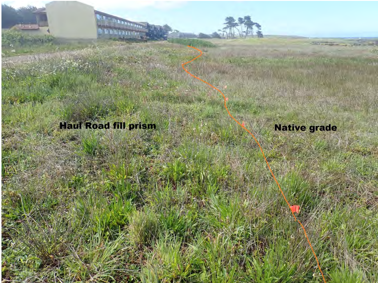
Figure 3. Haul road fill prism facing south.
