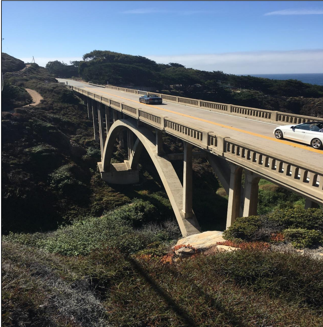
Figure 1-10 Photo of Garrapata Creek Bridge
