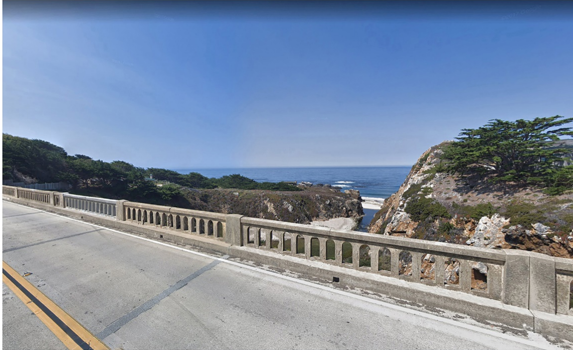
Figure 1-11 Photo of Existing Garrapata Creek Bridge Rail
