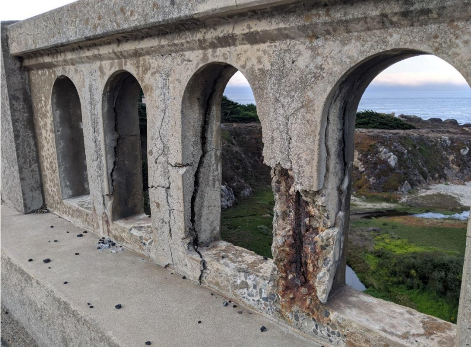
Figure 1-4 Photo of Garrapata Creek Bridge Rail Damage
