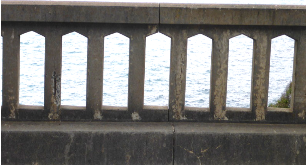
Figure 1-2 Photo of Bixby Creek Bridge Rail Deterioration
