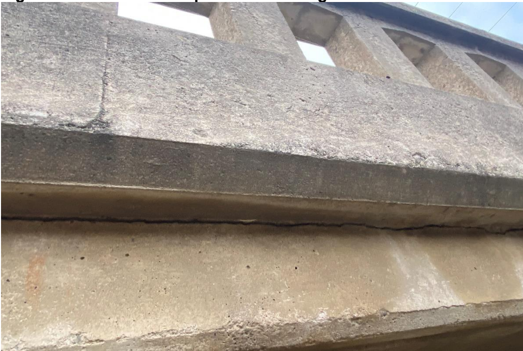
Figure 1-7 Photo of Malpas Creek Bridge Rail Deterioration
