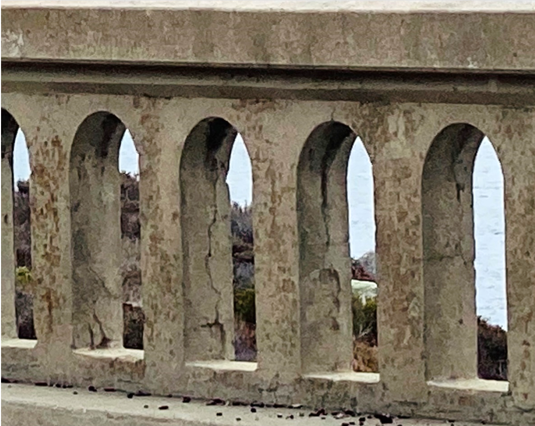
Figure 1-7 Photo of Malpas Creek Bridge Rail Deterioration
