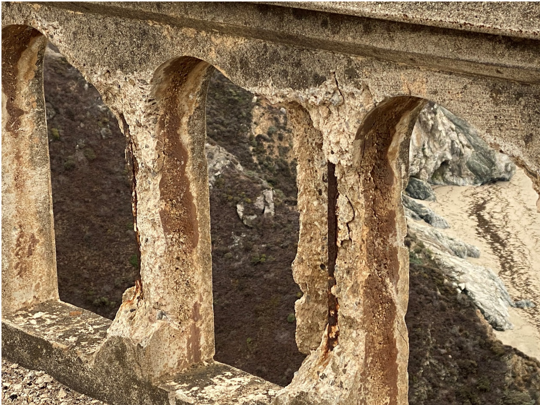
Figure 1-2 Photo of Bixby Creek Bridge Rail Deterioration
