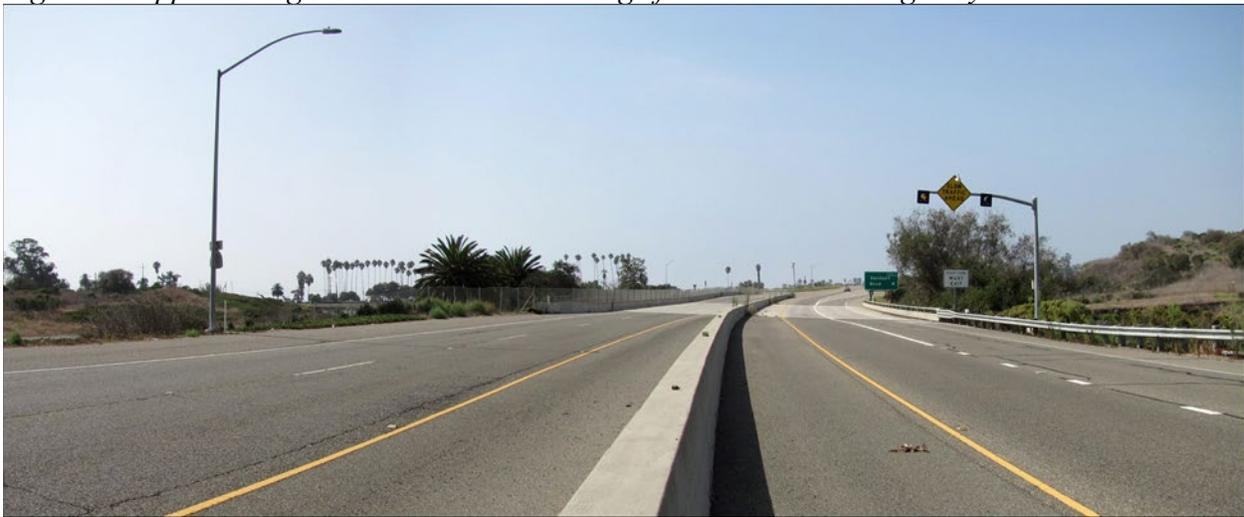
The existing four lane highway bridge structure is a seven span reinforced concrete slab bridge. Highway 217 is primarily a four-lane freeway with 12-foot wide lanes, 10-foot wide inside and outside shoulders with a continuous single concrete median barrier which results in a 22-foot wide median. At the project location Highway 217 changes from a four lane freeway to a two lane freeway.
