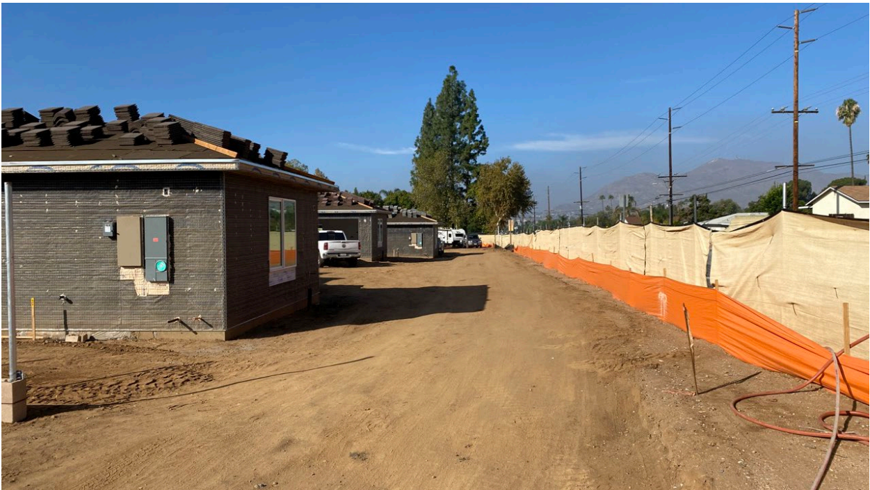
Photograph 6. MW-05a, eastern extent of project site facing west, entire location was under construction upon arrival.
