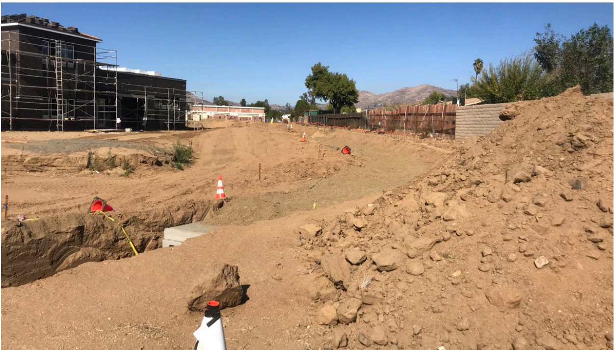
Photograph 14. MW-08b, entire parcel currently undergoing development during the time of surveys. View from southeast corner facing north.
