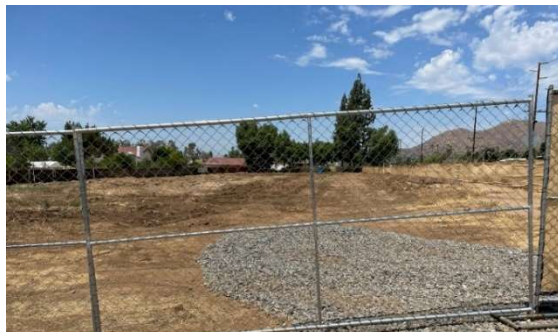
MW Site-5a: View west from Kilgore Street
