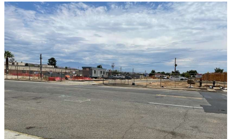
MW Site-8b: View site from Indian Street, currently under construction
