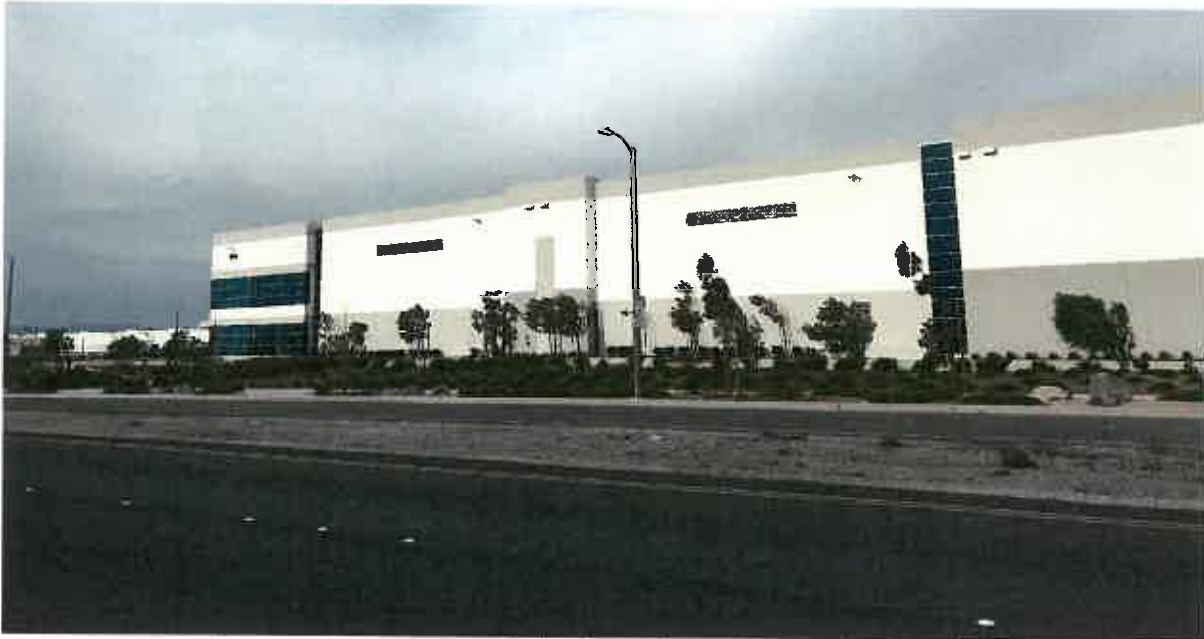
Although provided for illustrative purposes only, the image above shows how building faces visible from public roadways incorporate angular changes in massing, building materials, color, texture, and accents; no loading docks are to be visible from these roadways.
