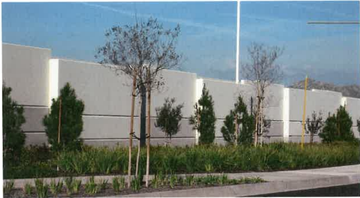
Although provided for illustrative purposes only, the image above conceptually shows concrete screen walls provided along public roadways to screen industrial uses from public views.
