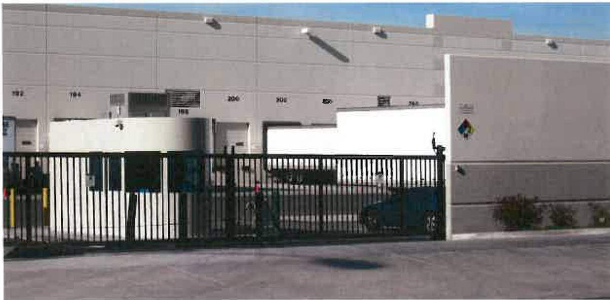
Although provided for illustrative purposes only, the image above shows screening and wall concepts for truck courts and loading docks.
