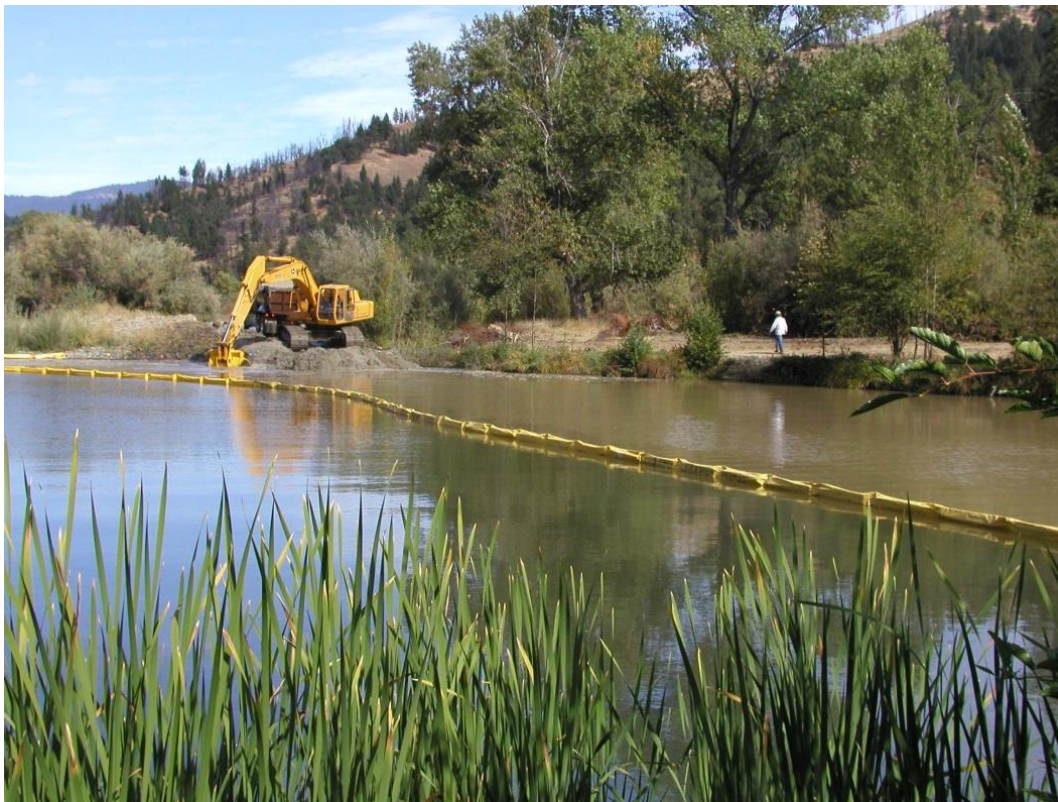
Figure 3. Upper Hamilton Pond dredge area, isolated from pond by turbidity curtain.
