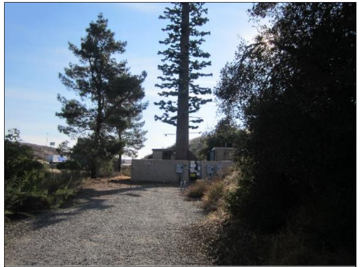
16. Cell tower facility adjacent northwest of the subject property.
