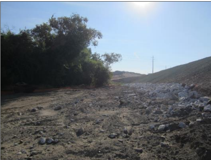
21. View east from the southwest corner of the subject property.
