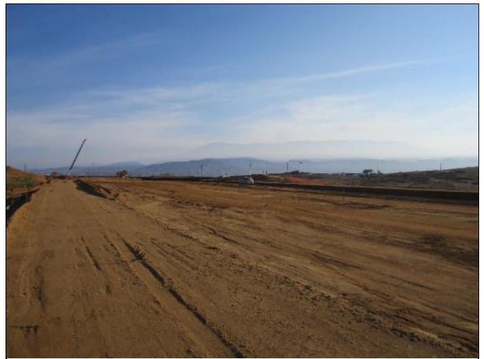
4. View of road grading adjacent east of the subject property.
