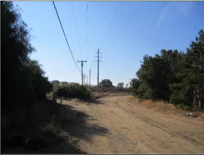
19. View south along west side of the subject property.
