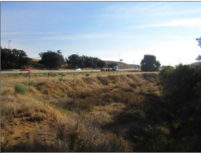
15. Highway 60 along north side of the subject property.
