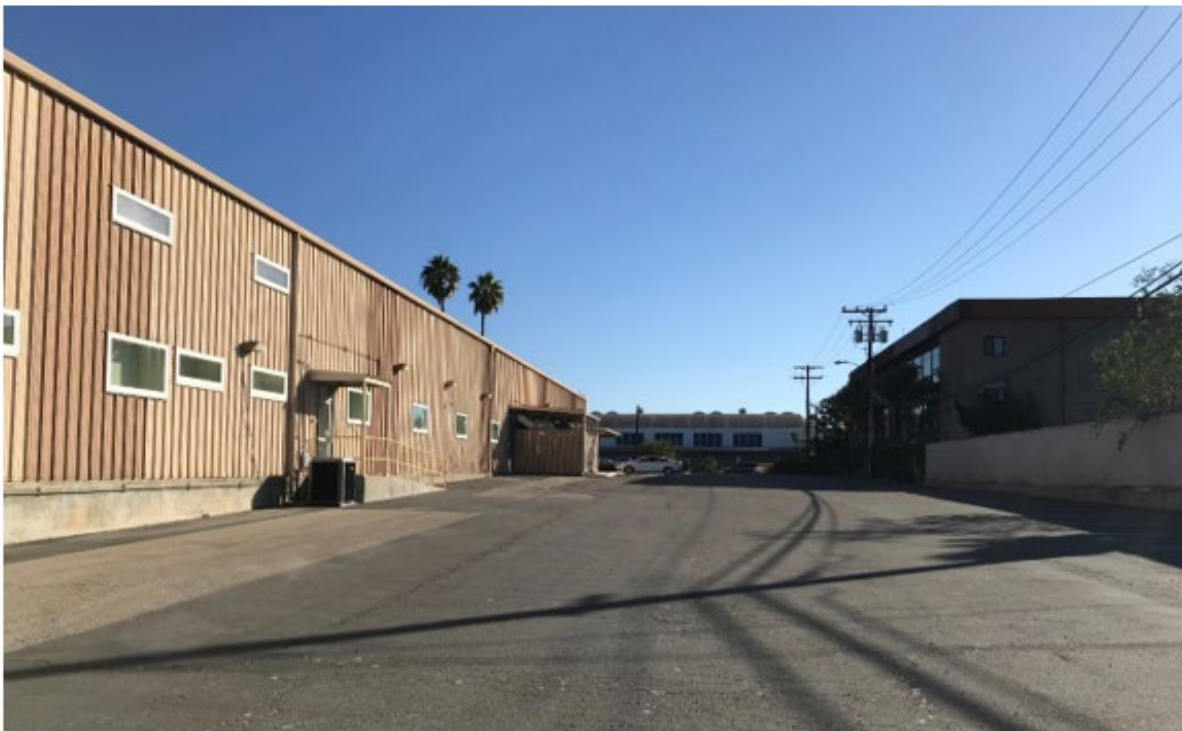
View of the south side of the existing building looking east towards S. Patera Lane
