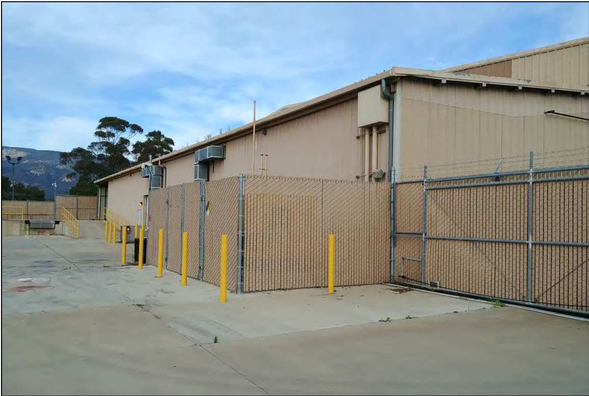
Figure 7 Enclosed Area at Rear of Building
