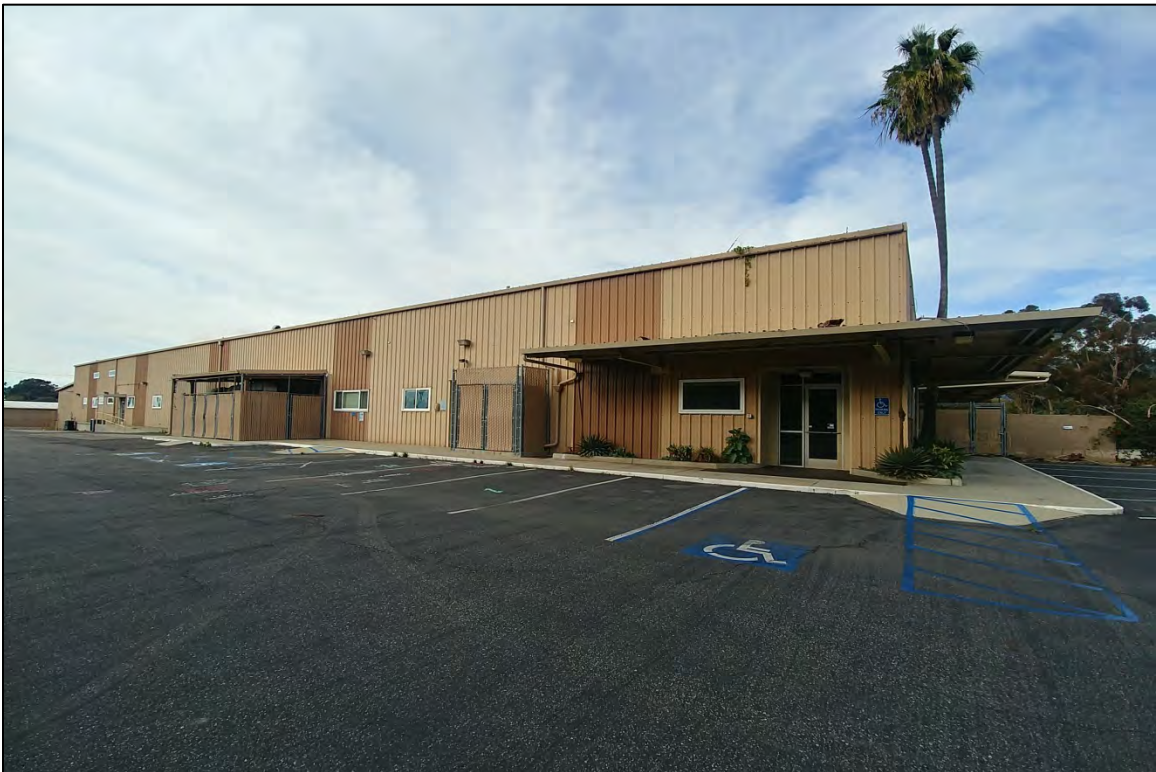
Figure 5 South Elevation and Primary Entrance at Corner
