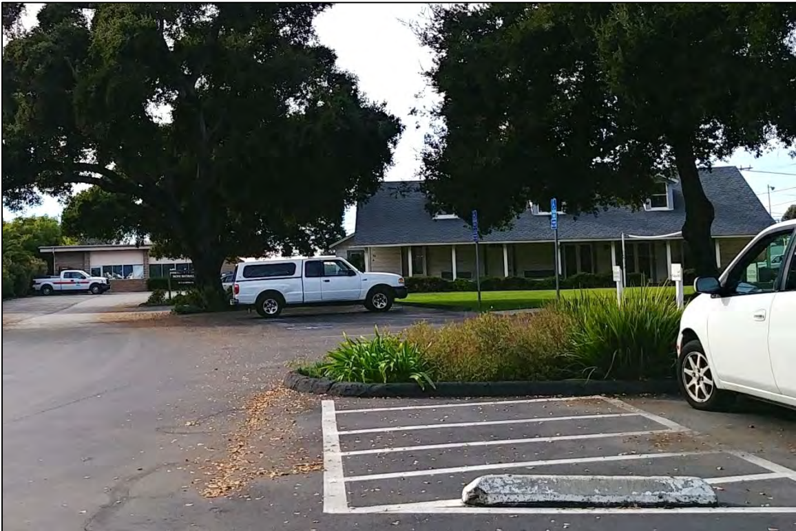
Figure 13 Hill Adobe, Parking Lot, and One-Story Office Building Constructed to the Rear
