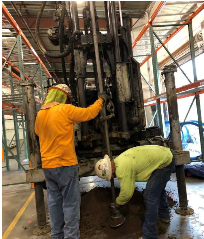
PHOTO 2.3.2-1: Boring Inside Existing Warehouse
