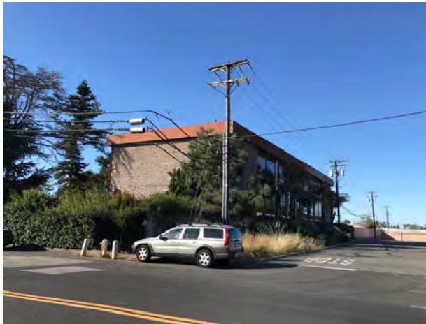
Photograph 11. View of the southern adjacent commercial office building and pole-mounted transformers (33 S. La Patera Lane), facing southwest.
