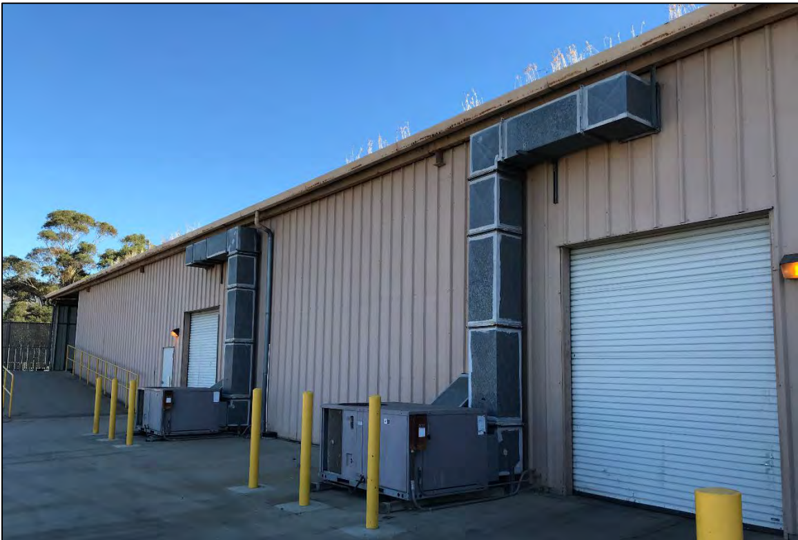
Figure 8 Closeup of West Elevation (Rear of Building)
