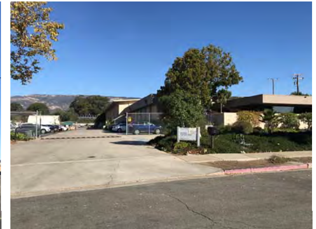
Photograph 12. View of the western adjacent commercial building (6338 Lindmar Drive), facing north.
