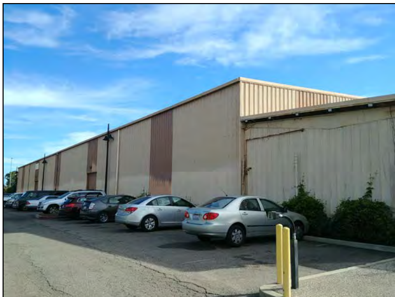
North elevation, view southeast.
