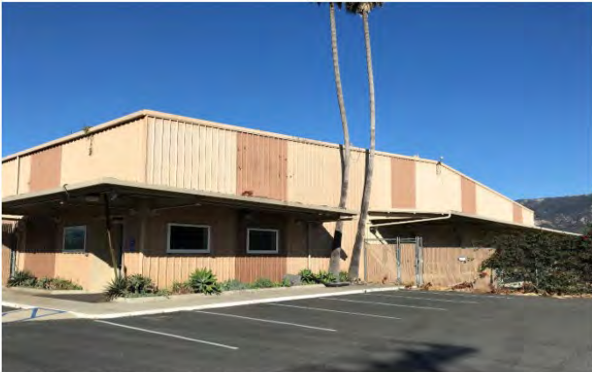
View of the east side of the existing building looking northwest
