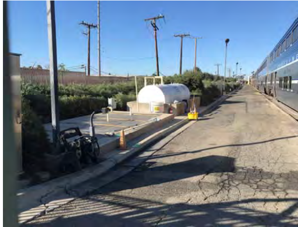
Photograph 8. View of the northwestern adjacent 3,000-gallon waste oil AST, facing west.
