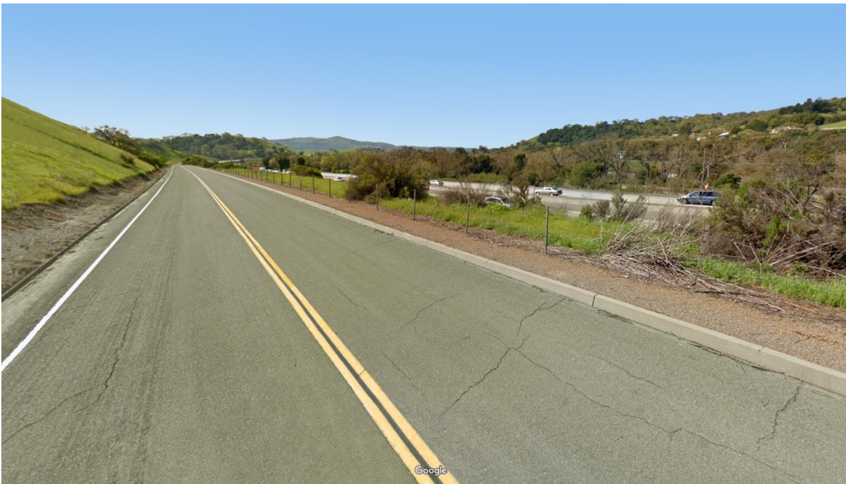
Figure 2.1.8-2a: Key View 1, Koopman Road Looking South Toward I-680, Existing Condition
