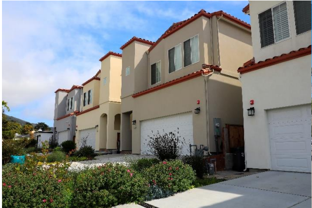
Single Family Residential Homes on B Street
