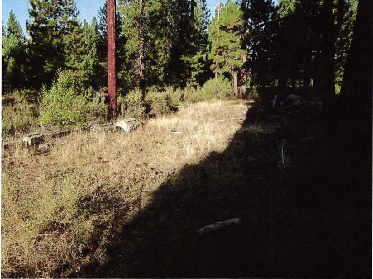
Photo 4: Concrete Footings from Foundation.
