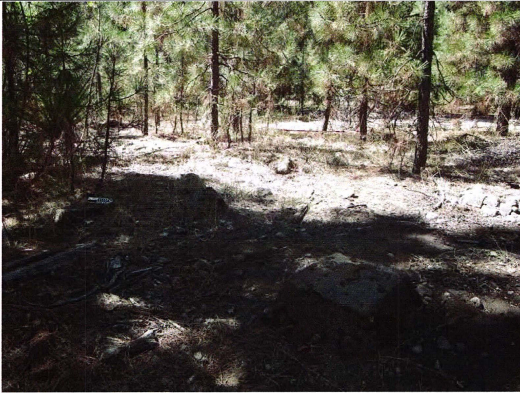
Photo 1: Overview of Foundation 2. View is southwest. Piers in lower right and middle left frame. Scale bar in background is 6'7".
