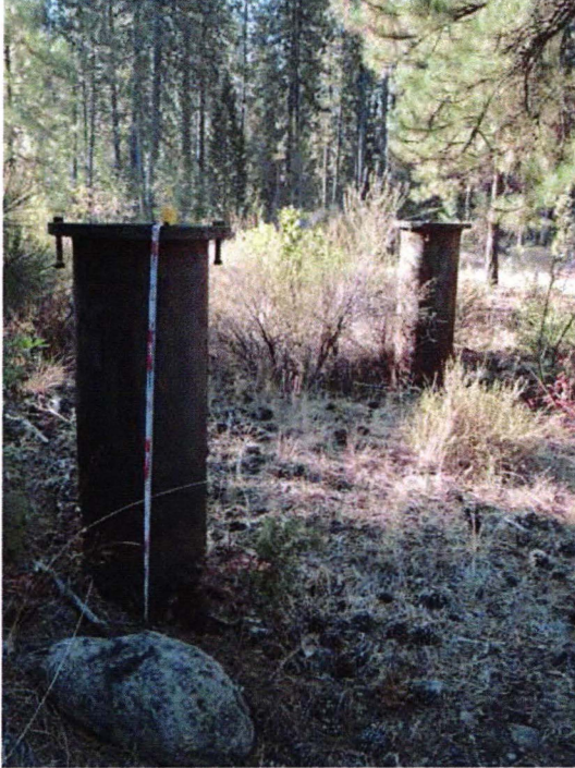
Photo 1: Pipes at Eastern Edge of Foundation.
