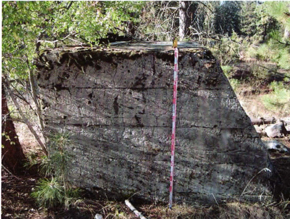
Photo 3: Triangular Board Form Footing.
