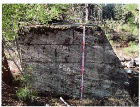
Photo 3: Triangular Board Forn1 Footing.
