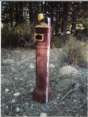
Photo 2. Scale showing height of post indicator valve (87cm / 2' IO")
