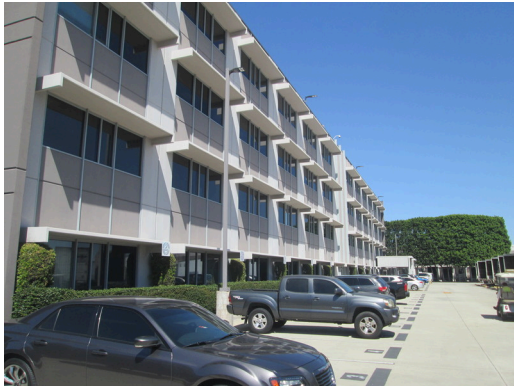
#3 SOUTH ELEVATION OF THE OFFICE BUILDING AT THE PROJECT
