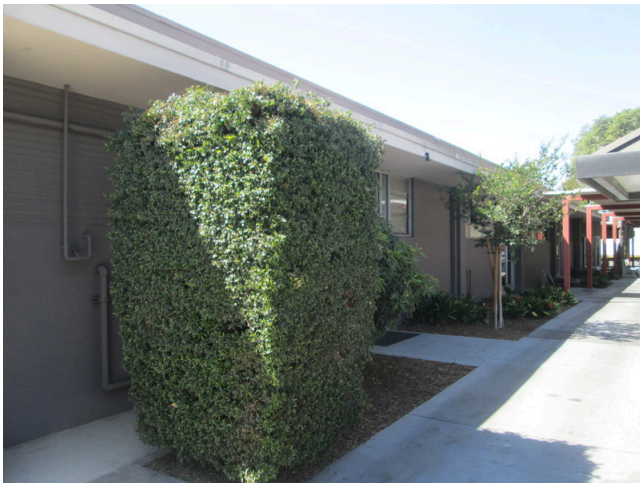
East elevation of the Cafeteria Building at the Project
