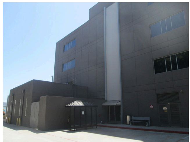
East elevation of the Office Building at the Project
