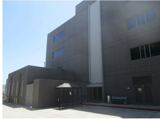
#2 EAST ELEVATION OF THE OFFICE BUILDING AT THE PROJECT
