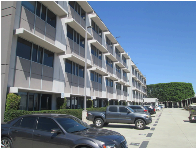
South elevation of the Office Building at the Project
