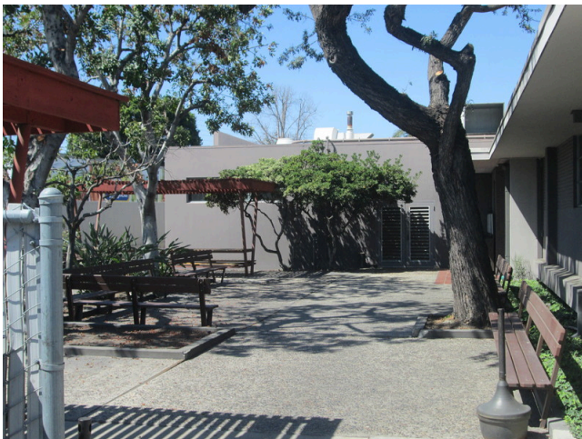
Outdoor patio and the southwest elevations of the Cafeteria Building at the Project
