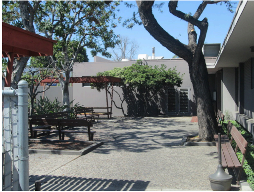
#7 OUTDOOR PATIO AND THE SOUTHWEST ELEVATIONS OF THE CAFETERIA BUILDING AT THE PROJECT
