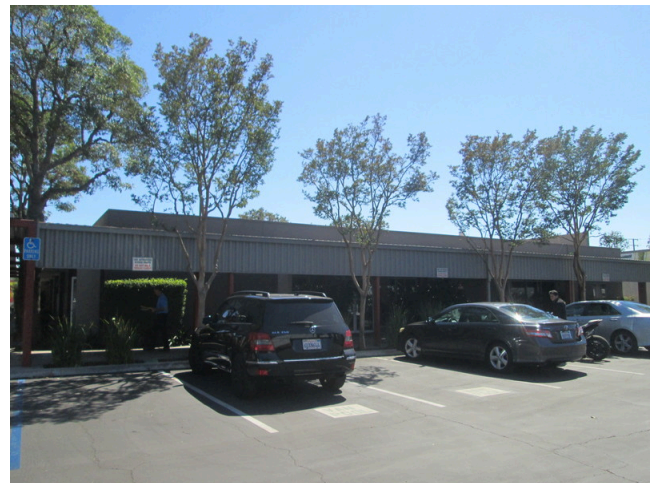
North elevation of the Cafeteria Building at the Project
