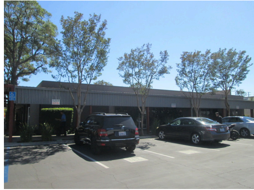
#8 NORTH ELEVATION OF THE CAFETERIA BUILDING AT THE PROJECT
