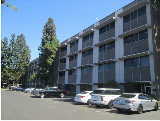
#1 NORTH ELEVATION OF THE OFFICE BUILDING AT THE PROJECT
