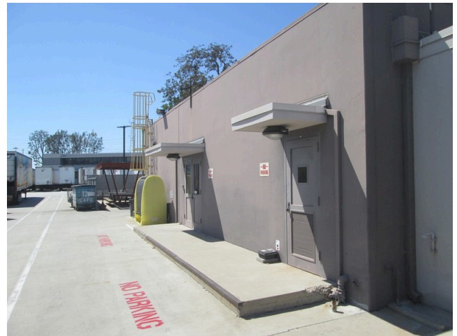
South elevation of the Cafeteria Building at the Project
