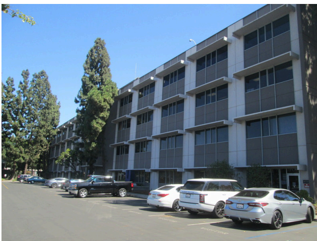
North elevation of the Office Building at the Project
