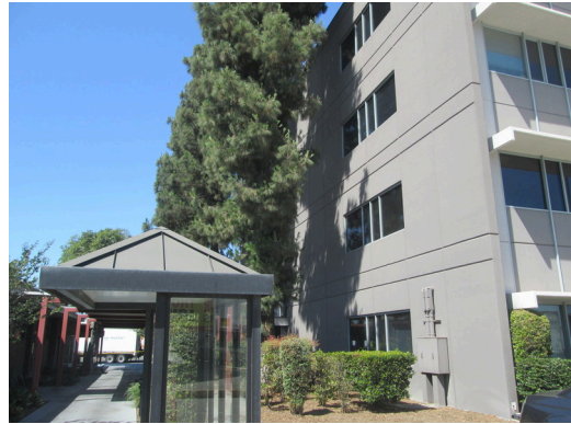
#4 CENTRAL COURTYARD AND THE WEST ELEVATION OF THE OFFICE BUILDING AT THE PROJECT
