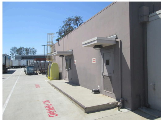
#6 SOUTH ELEVATION OF THE CAFETERIA BUILDING AT THE PROJECT
