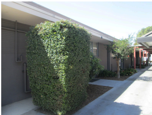
#5 EAST ELEVATION OF THE CAFETERIA BUILDING AT THE PROJECT
