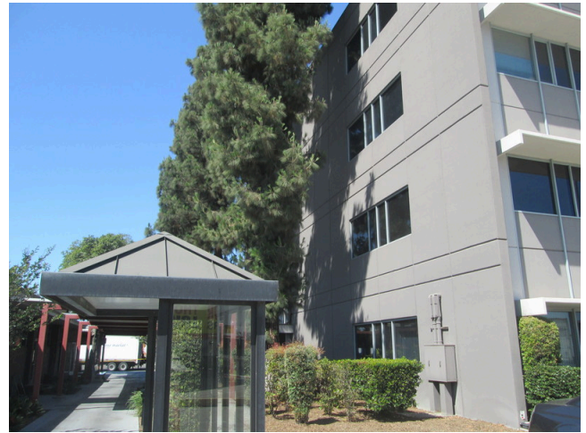
Central courtyard and the west elevation of the Office Building at the Project
