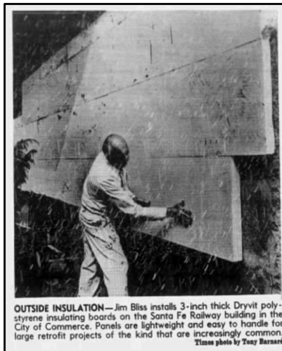
Plate 3.3–11: Application of the Dryvit panels to the “Santa Fe” office building in 1979. ( Photograph courtesy of Kinchen 1979b )
