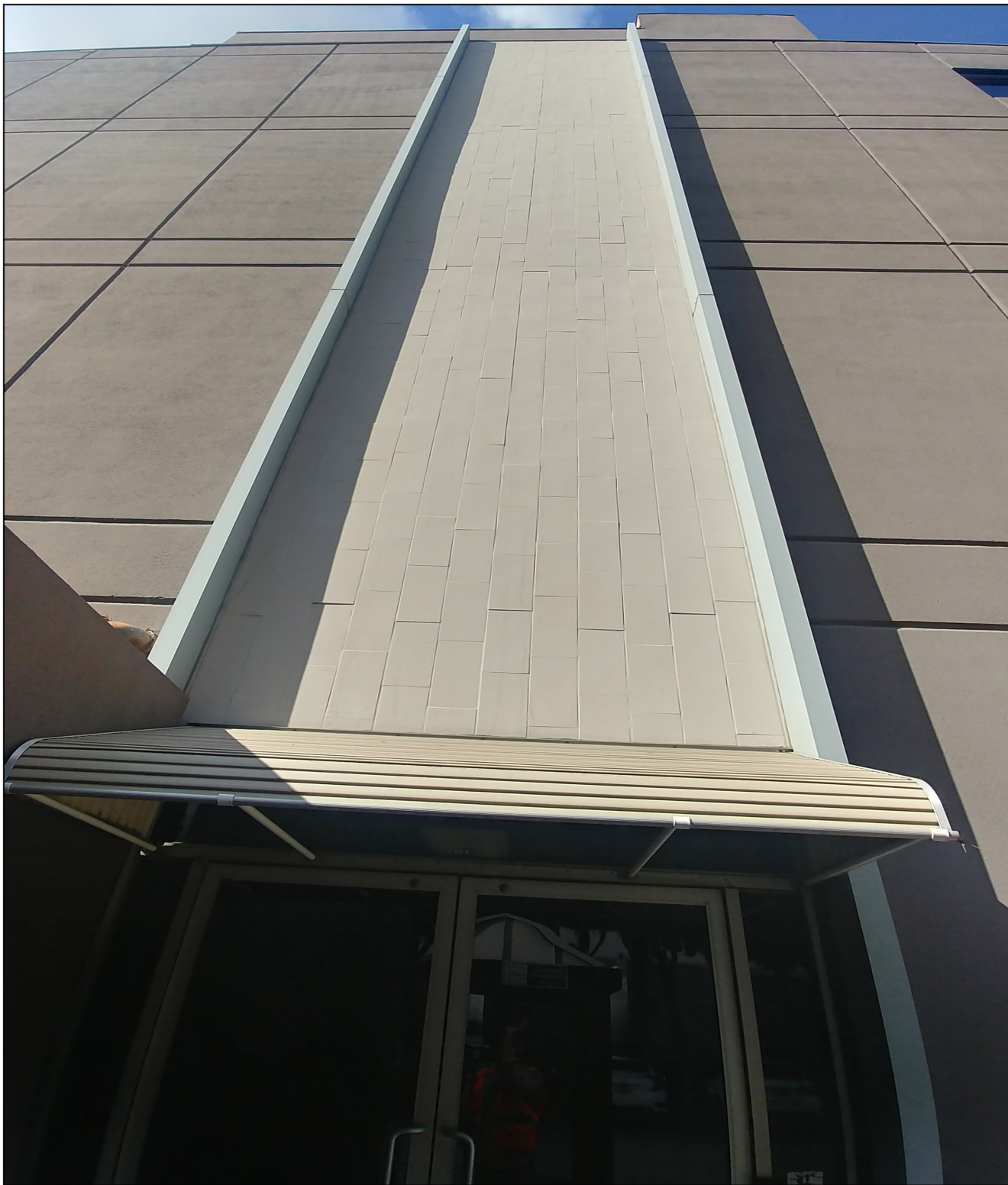
Plate 3.3–21 Close-Up View of the Ceramic Tile Veneer on the East Façade of the “Santa Fe” Office Building The Commerce Logistics Center Project
