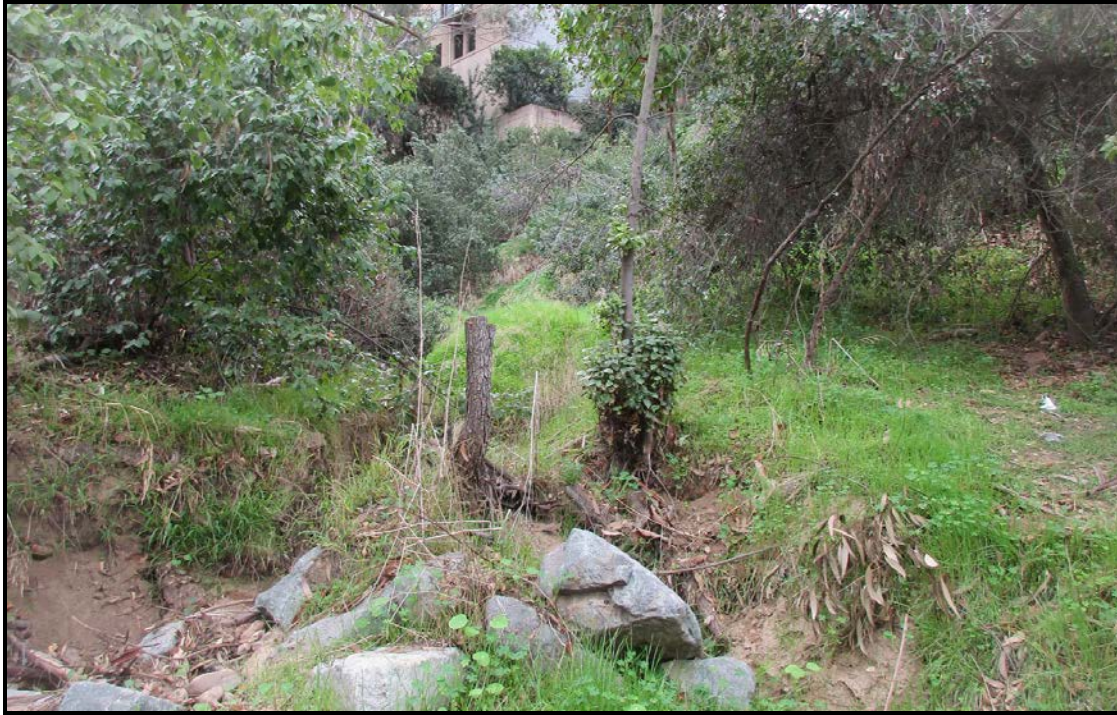
PHOTOGRAPH 4 Storm Drain toward First and Front Streets at the Low Point, Note Deep Erosional Cut
