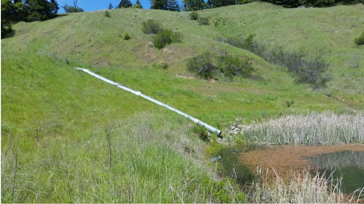
**Photo 3.** Culvert connected Upper Pond with Lower Pond
