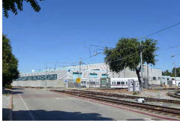
Figure 54. VTA Light Rail Facility.
