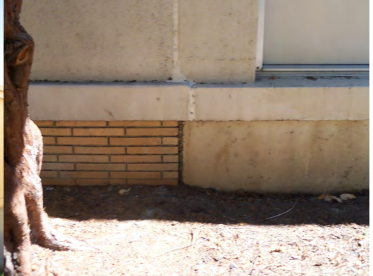
Figure 30. Cantilevered wall over foundation Source: KVP Architects
