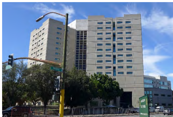
Figure 55. Santa Clara County Main Jail.
