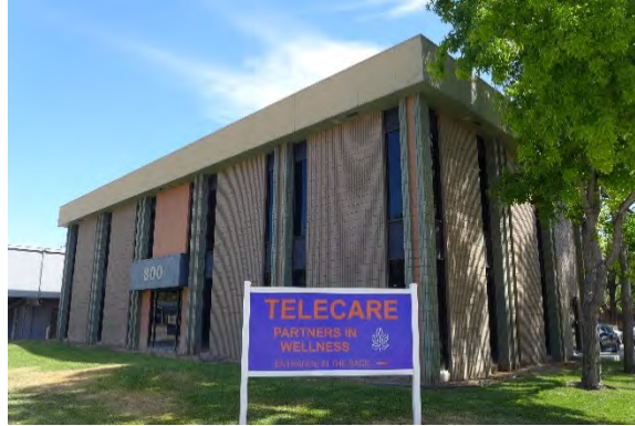
Figure 52. 800 N. First Street.
