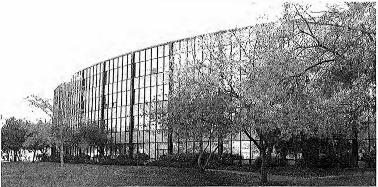
View of rear wall of office wing – facing southeast
