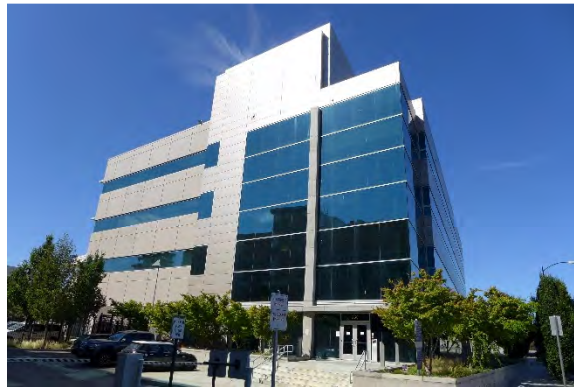
Figure 58. Santa Clara County Laboratory at 250 W. Hedding Street.
