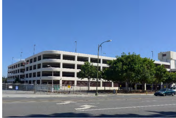
Figure 57. Civic Center Parking Garage.
