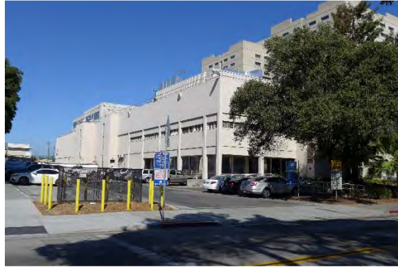
Figure 7. The Main Jail South.
