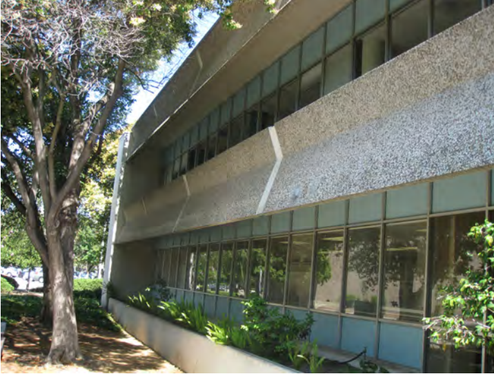
Figure 33. Cast concrete balconies and parapets Source: KVP Architects
