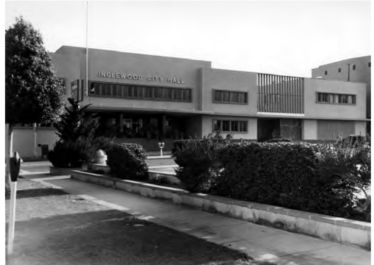
Figure 64: 1954 Inglewood City Hall Source: Inglewood Public Library
