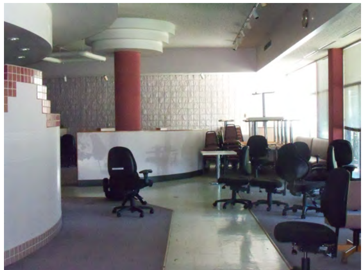
Figure 17. Cafeteria on first floor of wedge wing Source: KVP Architects
