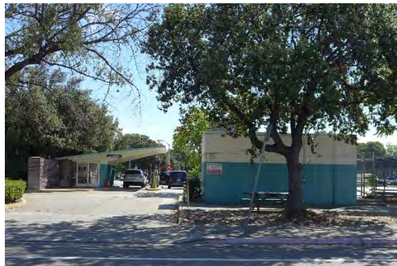
Figure 13. Service Garage and Gas Station.
