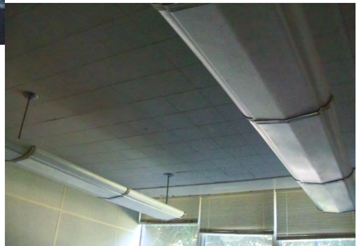
Figure 14. 1990s era office spaces on first floor Source: KVP Architects
