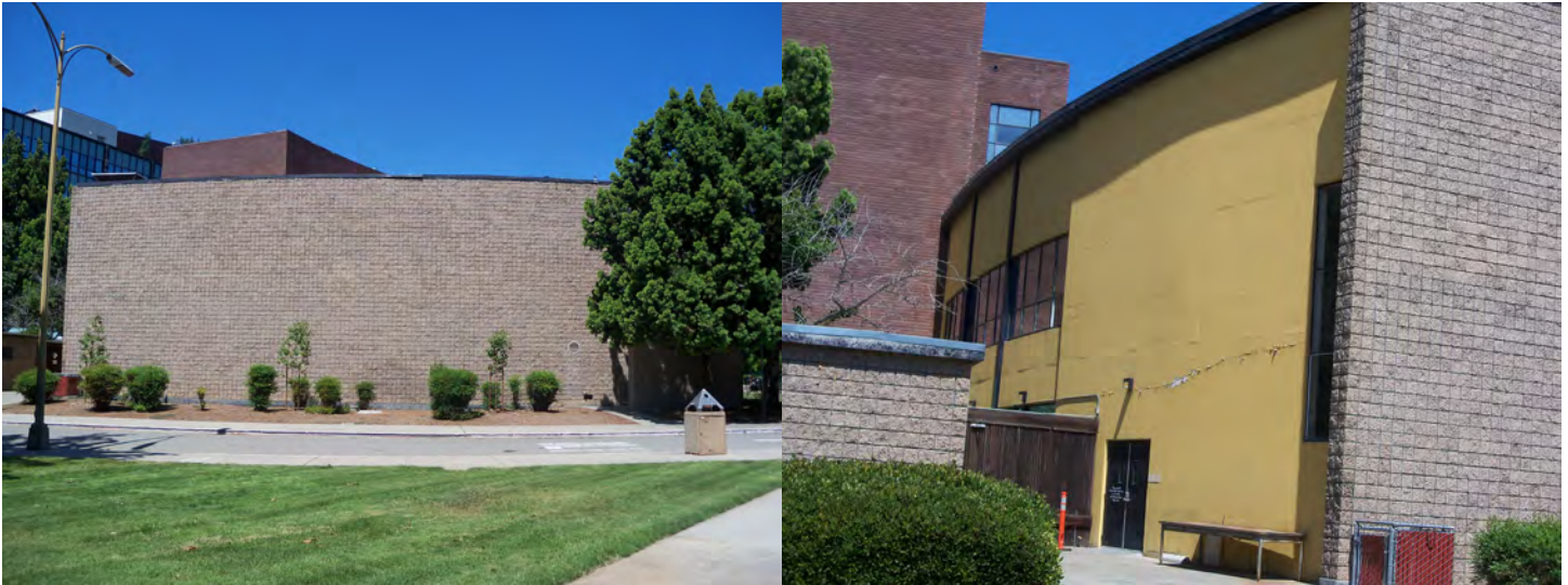
Figure 6. Concrete block facing on cafeteria/Council Chambers wing Source: KVP Architects
