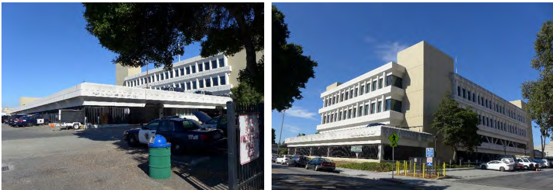
Figures 21 and 22. The Police Garage (left) and the Office of Emergency Services (right) buildings.
