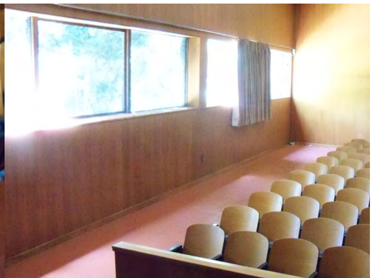
Figure 21. Windows on south wall of Council Chambers Source: KVP Architects
