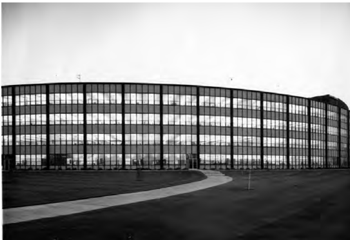
Figure 42. North side with concrete path c1960s Source: Sourisseau Academy for State and Local History
