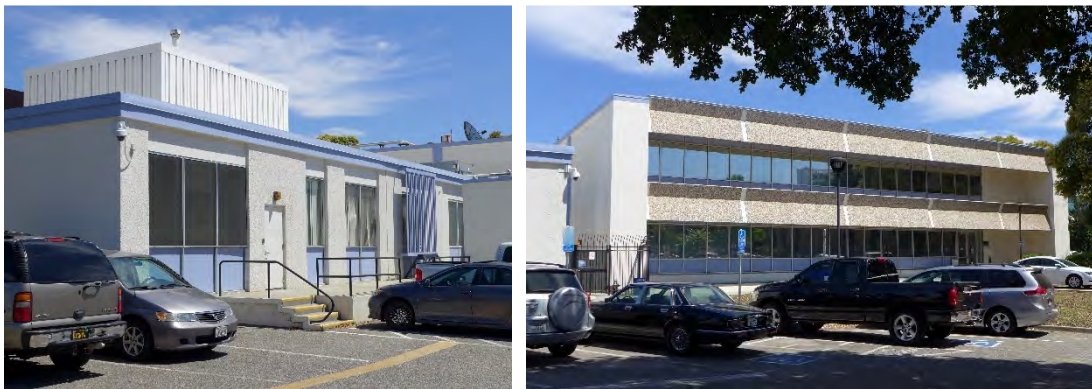
Figures 5 and 6. The original Health Building (left) and its later additions (right).
