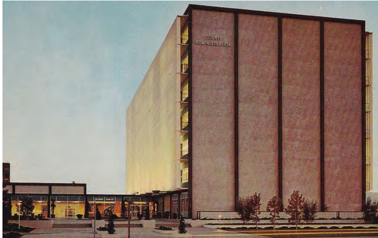
Figure 12. Santa Clara County Administration Building. 45
