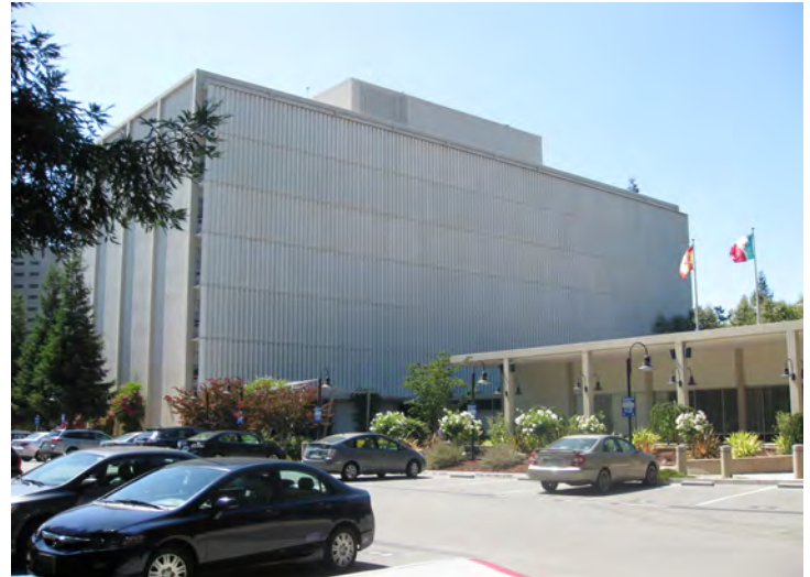
Figure 66. Current view of Original Santa Clara County Administration Building Source: KVP Architects
