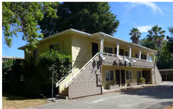
Figure 37. The apartment building at 954 N. First Street.
