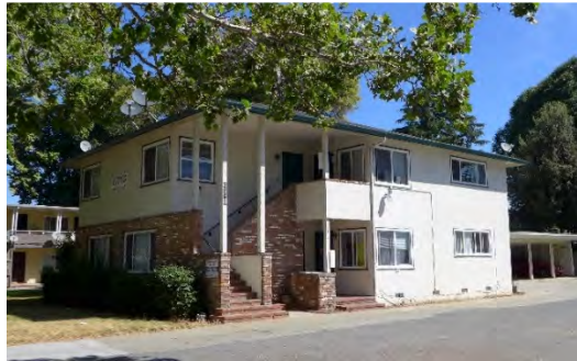
Figure 38. The apartment building at 940 N. First Street.
