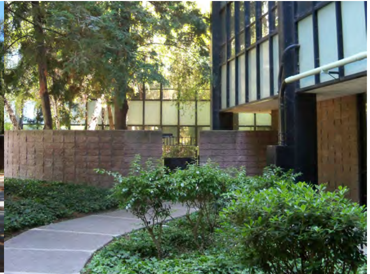
Figure 24. Exterior split face concrete block garden wall Source: KVP Architects
