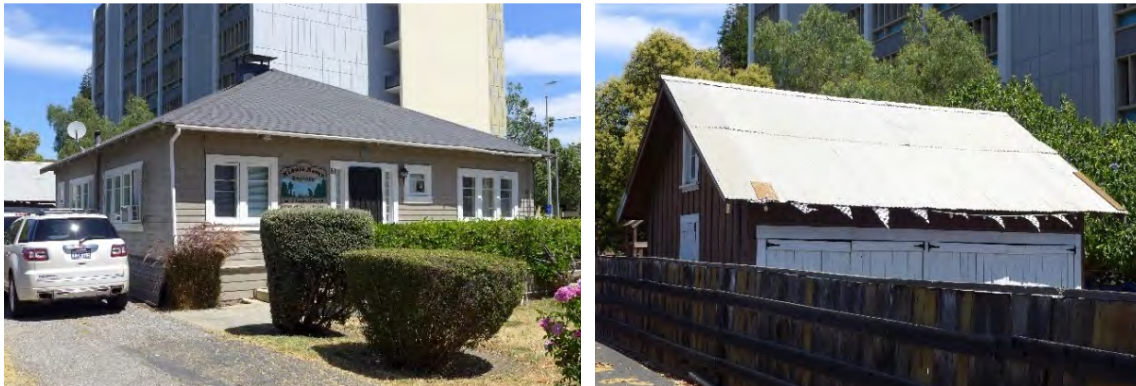
Figures 31 and 32. 61 Asbury Street, the house (left) and the outbuilding (right).
