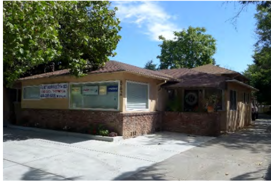
Figure 42. The front façade of 858-864 N. First Street.
