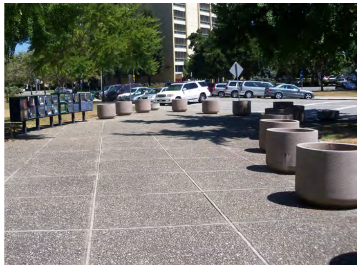
Figure 38. Decorative pebble aggregate concrete pathways at the former San José City Hall Source: KVP Architects
