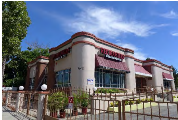
Figure 51. The restaurant building at 840 N. First Street.
