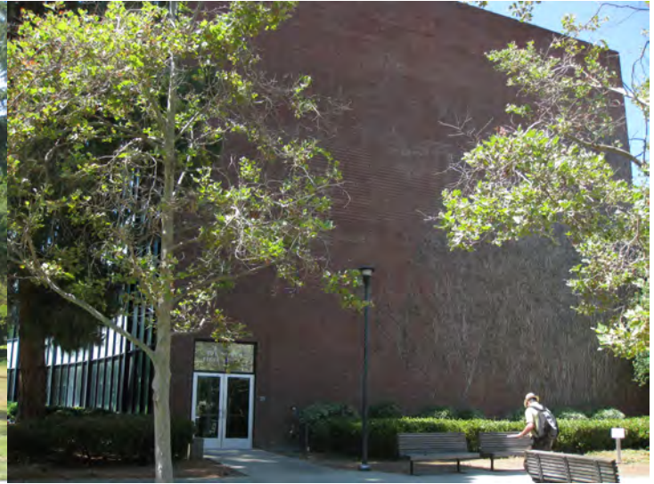
Figure 4. Brick veneer on west façade Source: KVP Architects
