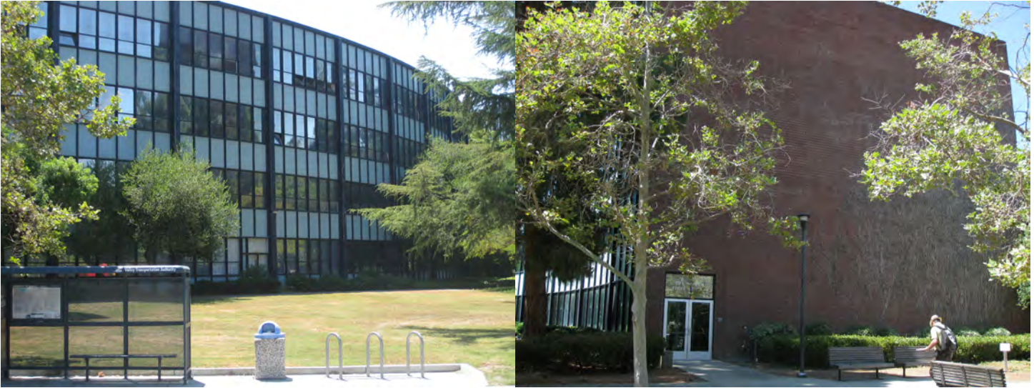
Figure 3. Curtain wall of glass and enamel panels on north façade Source: KVP Architects
