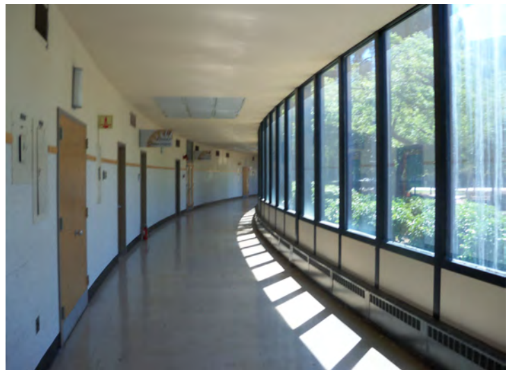
Figure 11. First floor corridor (typical) Source: KVP Architects
