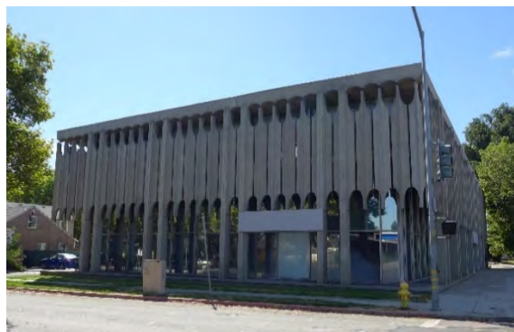
Figure 36. 990 N. First Street.
