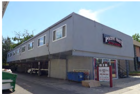
Figure 45. 816 N. First Street.
