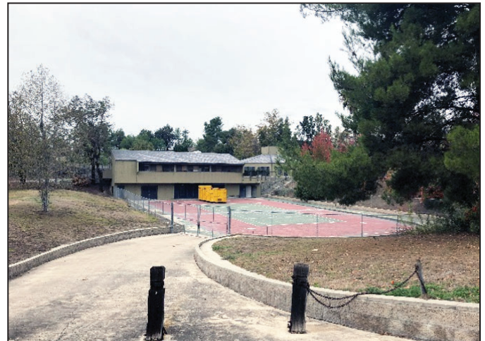
6. View looking north from the southern end of the property.
