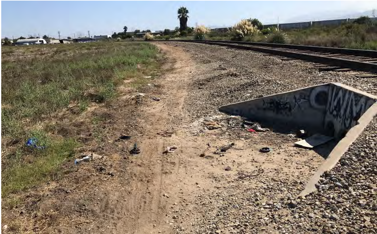
Photograph 6. Railroad track culvert (aspect: west, date: 09/17/19)
