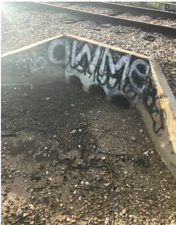
Figure 1- Existing Culvert Inlet
