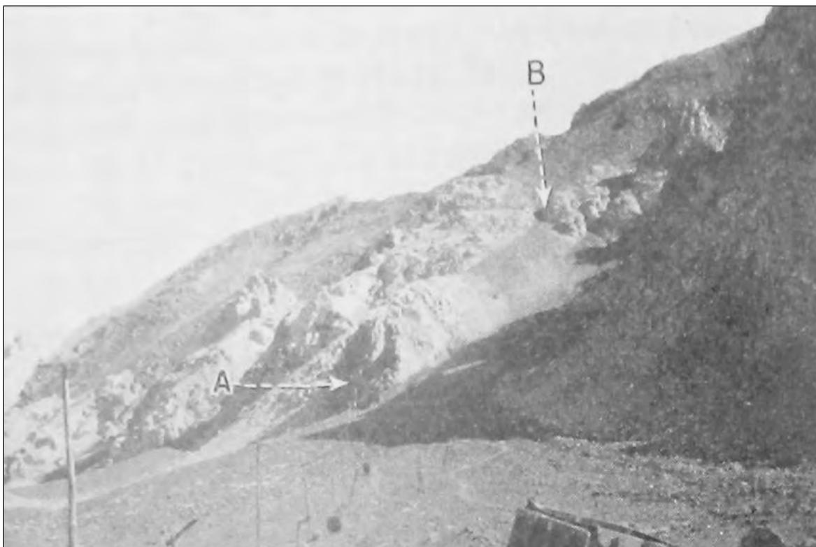
**Figure 10.** Outcrop of Tungsten deposit, showing upper and lower adits at B and A (Photograph from *Engineering and Mining Journal*, 10 April 1926:606).
