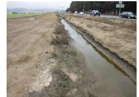
⑥ Drainage ditches at western end of project site (2017)
