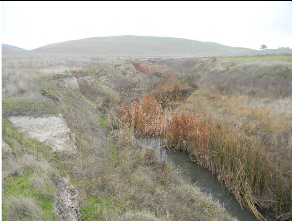
8. Photograph from the south of Arroyo Las Positas' deeply incised channel.
