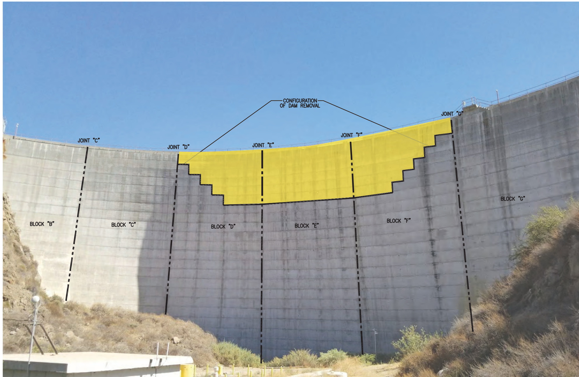
PHOTOGRAPH OF ARCH DAM DOWNSTREAM FACE NTS
