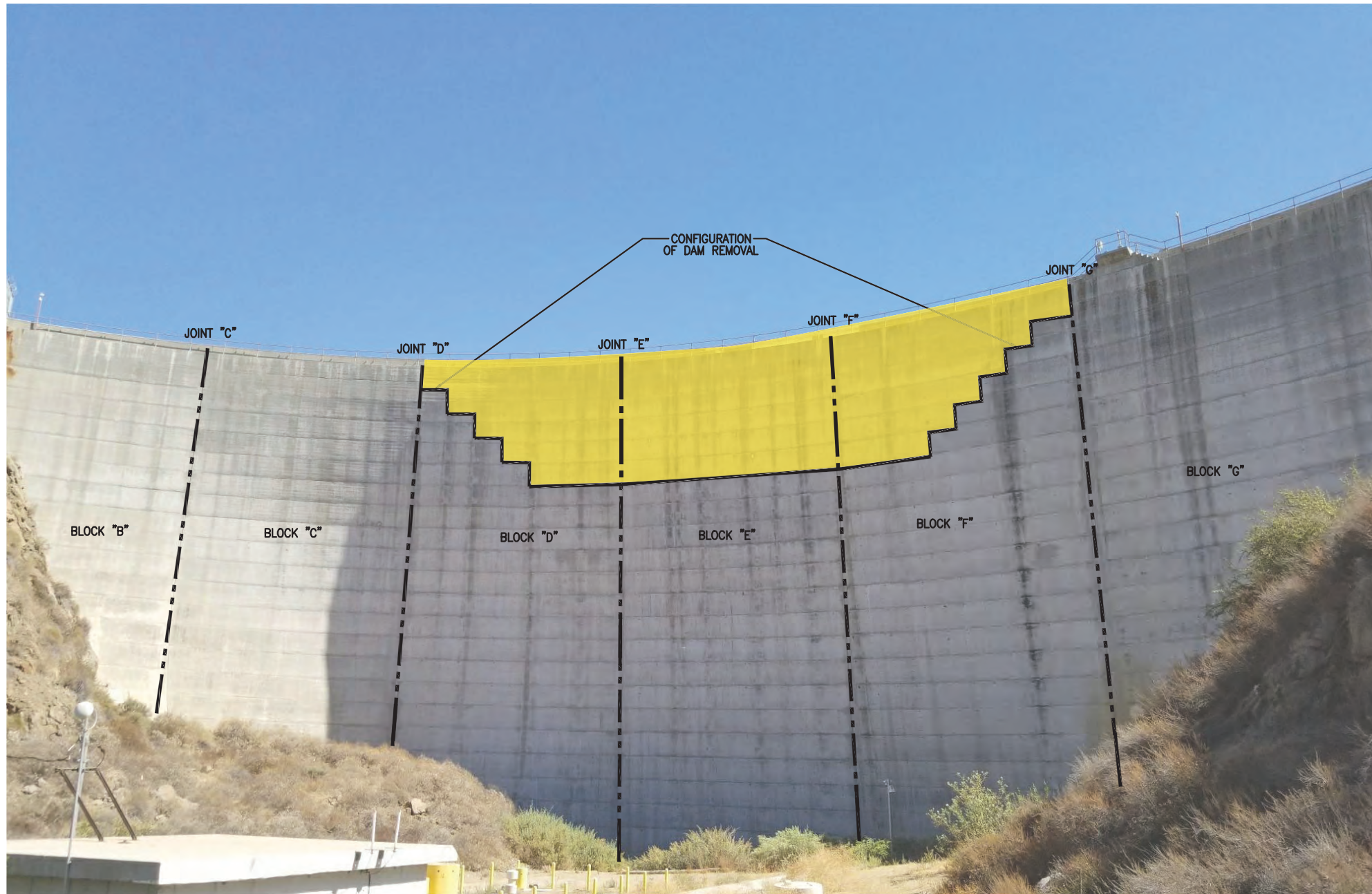
PHOTOGRAPH OF ARCH DAM DOWNSTREAM FACE NTS
