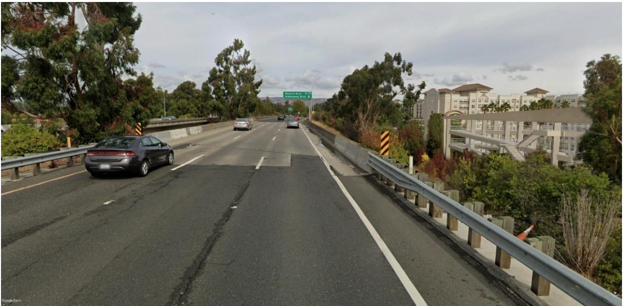
Figure 3.2-10. Viewpoint B – Four Corners Commercial Center from SR 84, looking northeast (Proposed Project)
