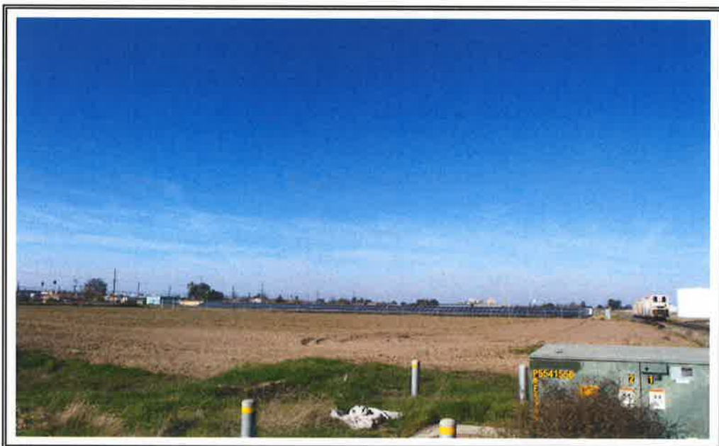
4. View of the Subject Property Looking Northwest Showing a Pad-Mounted Transformer and the Solar Array Adjoining to the North
