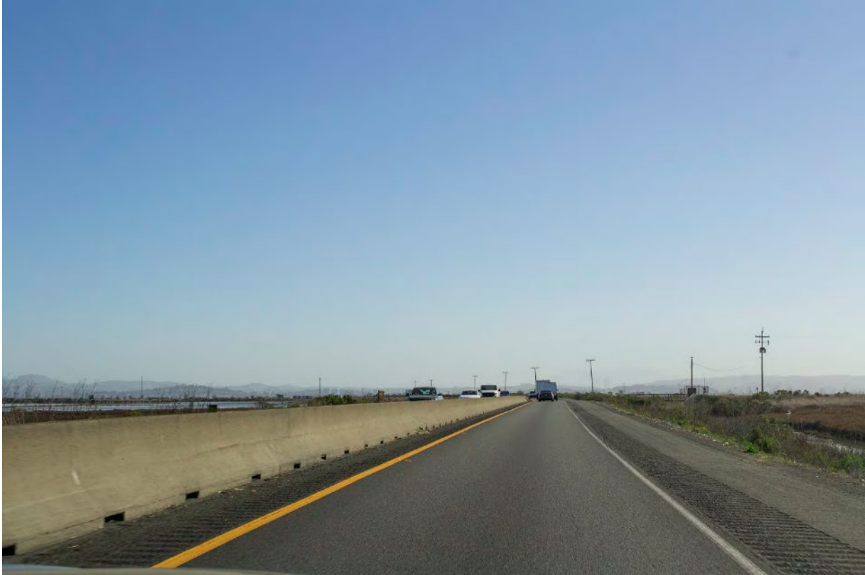
Figure 2-8 Existing Condition KV-3
