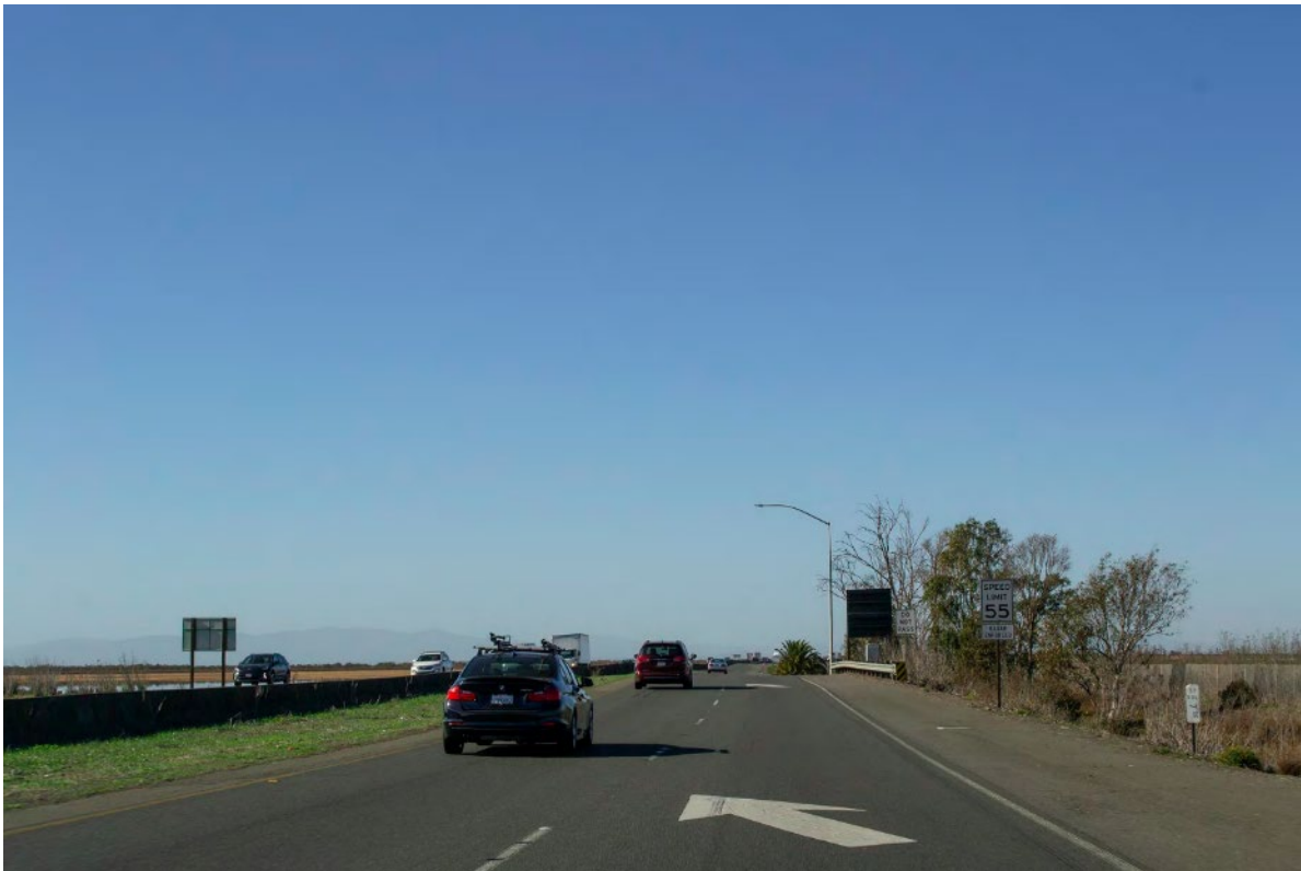
Figure 2-1 Existing Conditions from KV-1
