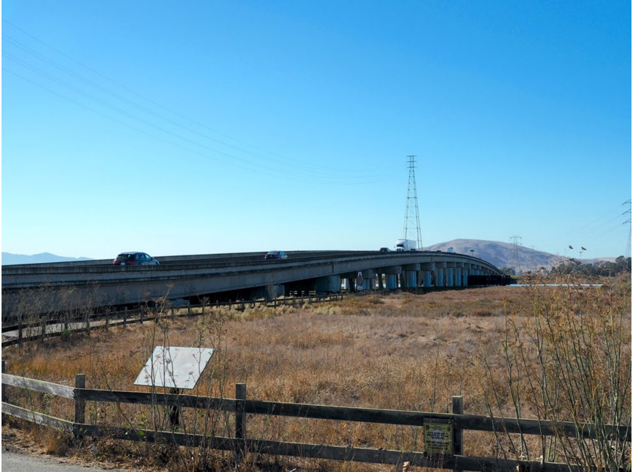
Figure 2-12 Existing Condition KV-4
