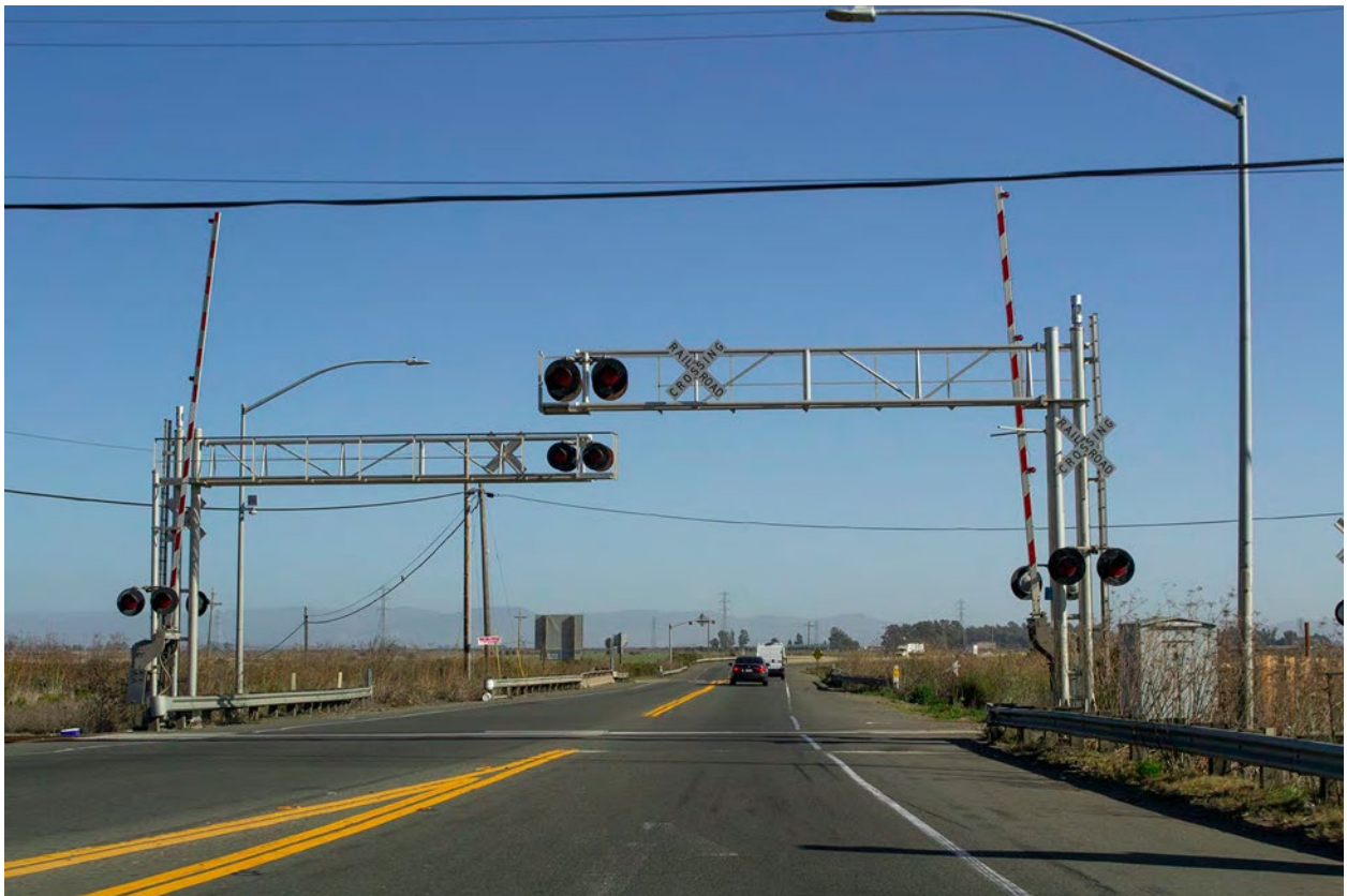
Figure 2-13 Existing Condition KV-5
