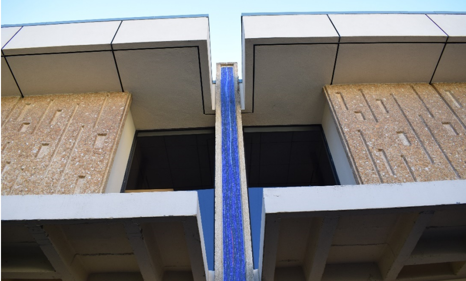
Figure 4. Detail of decorative gemstone mosaic and exposed aggregate panels with vertical scoring, Feb. 12, 2020. Source: ICF.
