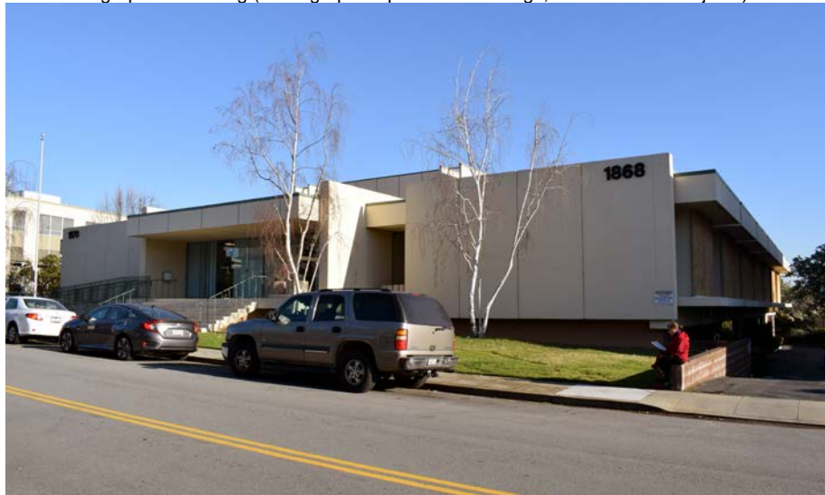
P5a. Photograph or Drawing (Photograph required for buildings, structures and objects)
