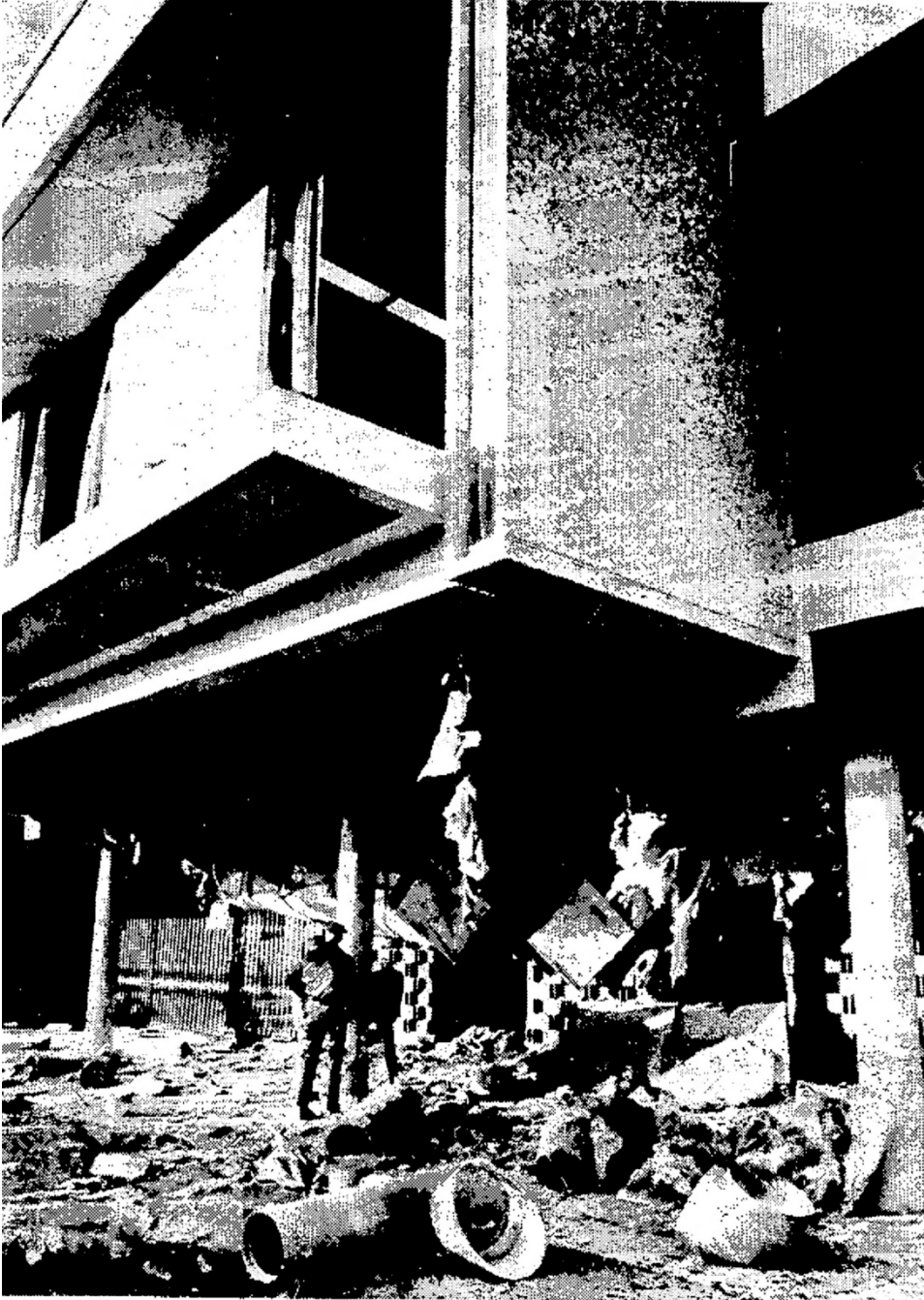
Figure 10. A few of the north (rear) façade of 1868-1870 Ogden Drive showing the damage cause by a bomb that detonated in April 1974. Source: The Times [San Mateo], April 18, 1974.
