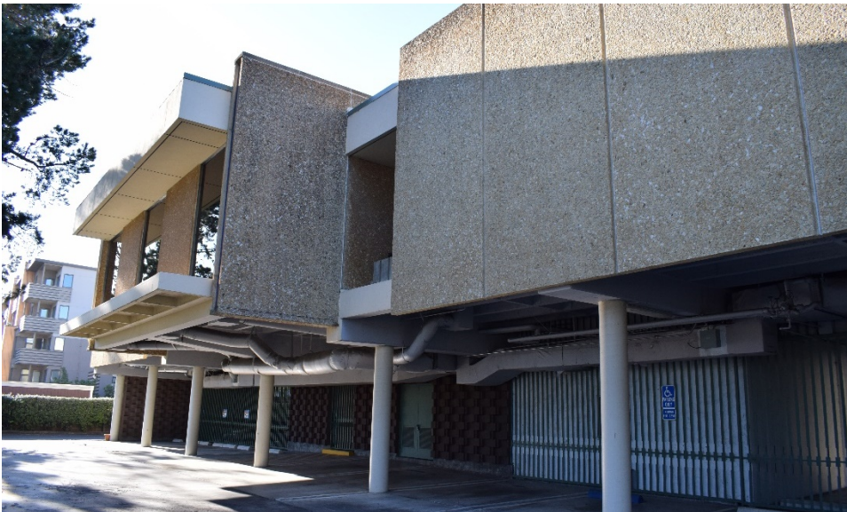
Figure 5. View of north facade, looking south, Feb. 12, 2020. Source: ICF.
