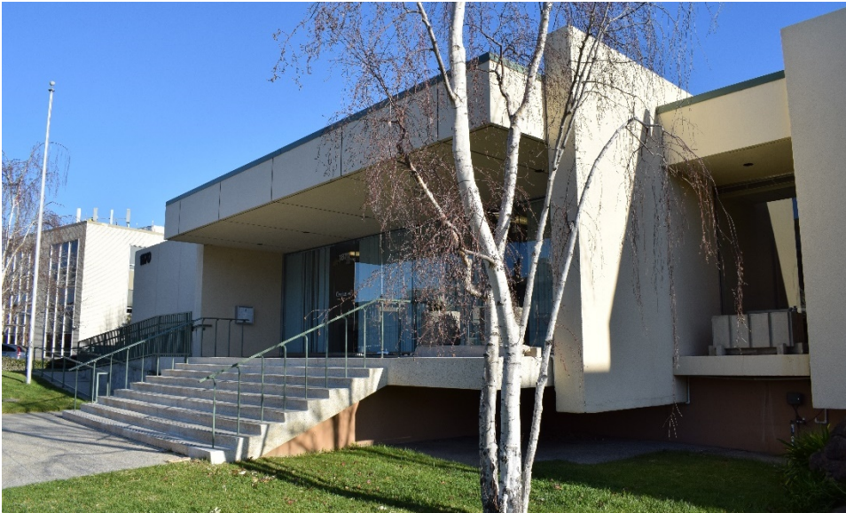
Figure 2. View of south (primary) façade of 1868-1870 Ogden Drive looking north, Feb. 12, 2020. Source: ICF.
