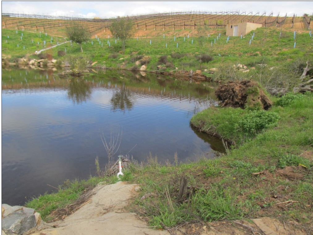
Photo 12. View of manmade seasonal pond 3, looking north, showing the V-ditch built to convey runoff and sediment from the vineyard (which was previously an orchard) into the pond. Visible on the right is a tree that had recently toppled over, likely due to unusually wet soil conditions. Photo taken February 28, 2019.
