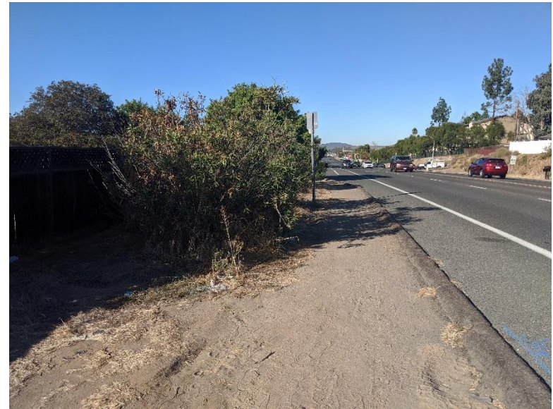
Photograph 3 – South side of Mapleview Street, facing west towards pavement improvement area.
