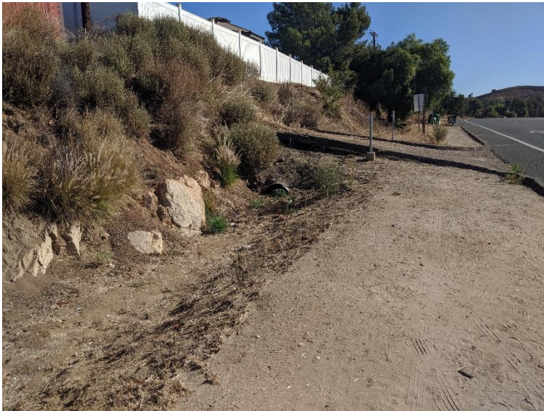
Photograph 5 – North side of Maplevue Street, facing east towards the pavement improvement area
