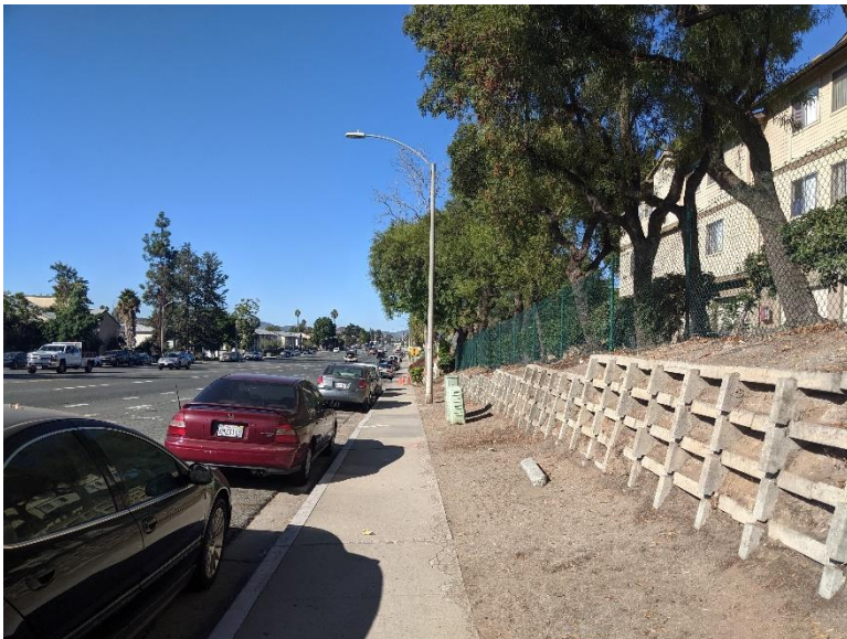
Photograph 6 – North side of Maplevue Street, facing west towards the gutter improvement area
