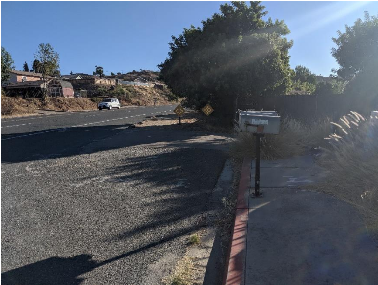
Photograph 1 – South side of Mapleview Street, facing east towards pavement improvement area.
