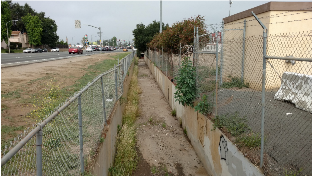
Photograph 1 – Concrete-lined ditch north of Mapleview Street, facing west.
