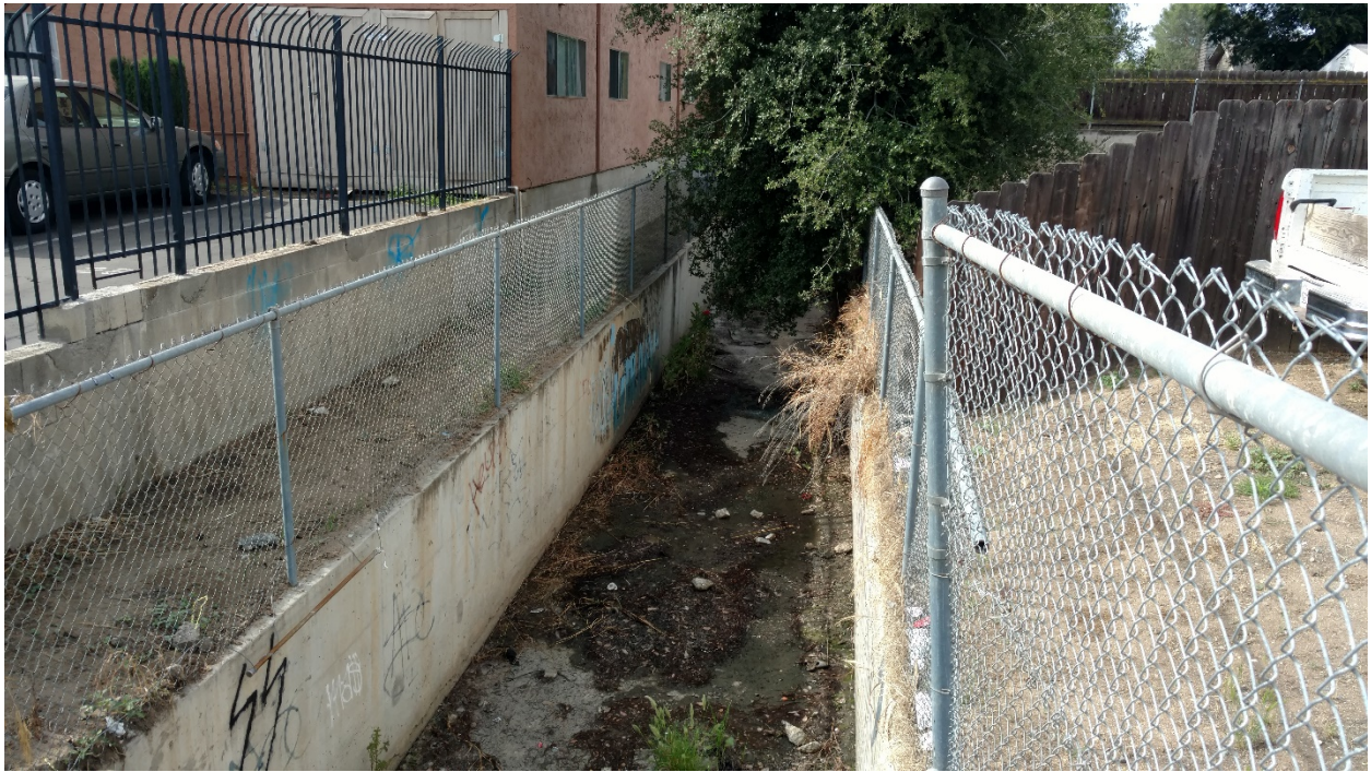
Photograph 2 – Concrete-lined ditch south of Mapleview Street, facing south.
